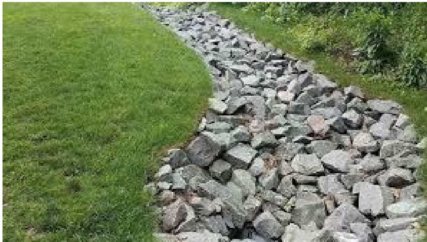
Image 3-4 Stone-lined Swale
