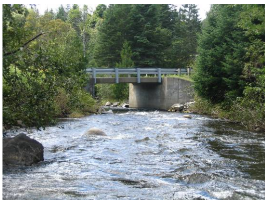
Figure 6. Undersized bridge with poor alignment in R30B
