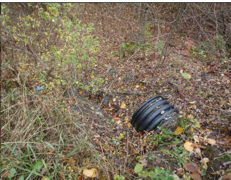
Photo 2. Elevated and eroding culvert outlet
