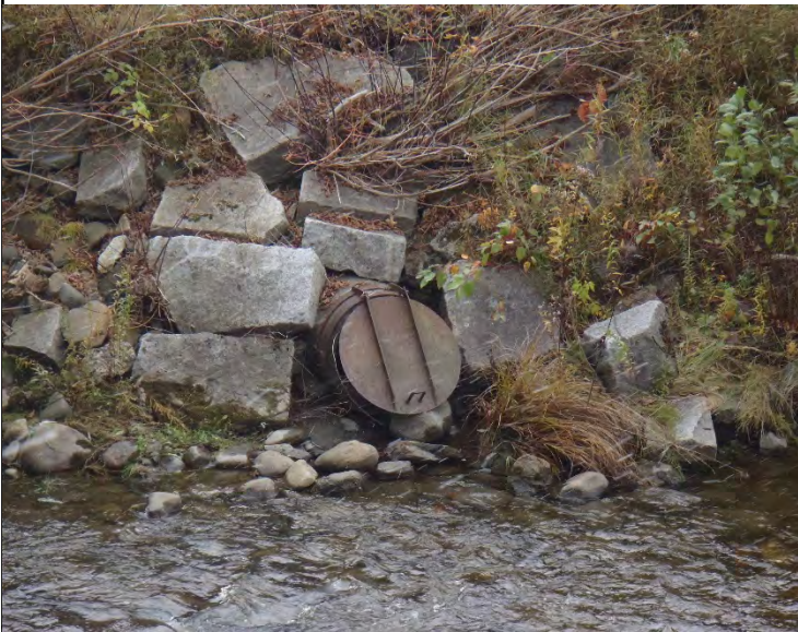
Photo 1. Existing culvert outlet with trash can style outlet structure
