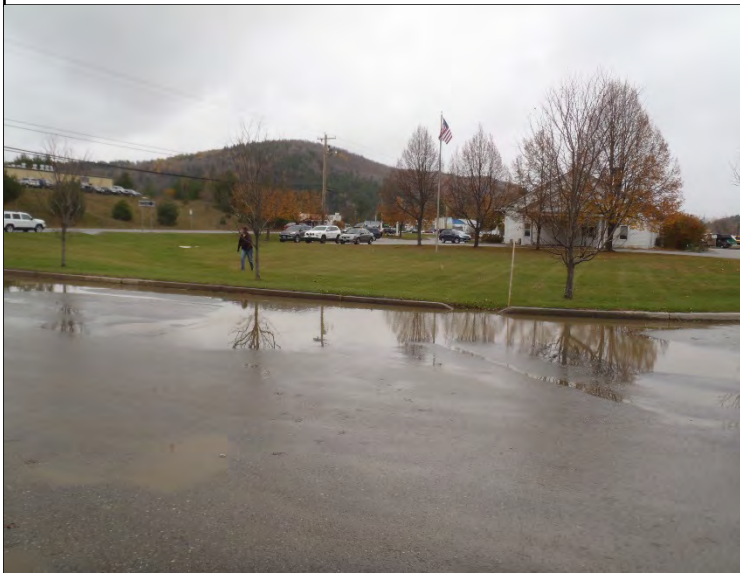
Photo 1. Ponding water due to settling and/or plugged or damaged drainage infrastructure
