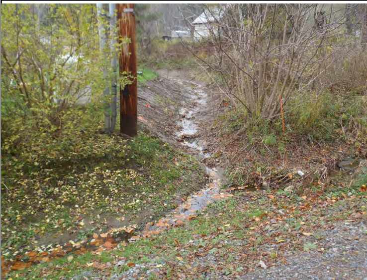
Photo 1. Destabilized open ditch lacking erosion control
