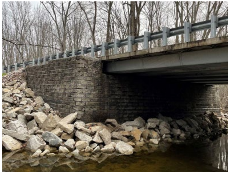
Image 3-6 Stone Stabilization
