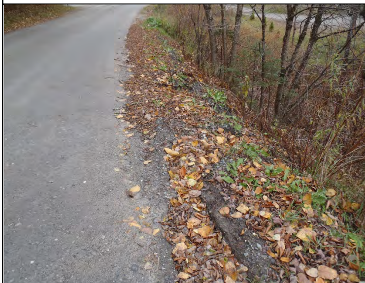
Photo 1. Shoulder berm/erosion and gully formation
