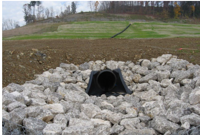
Image 3-2: Outfall Stabilization
