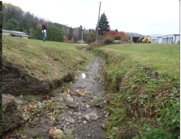
Photo 2. Erosion within drainage channel
