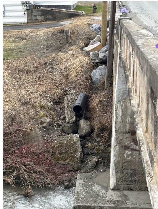
Image 2-3: Erosion on Northwest Side of Main Street Bridge
