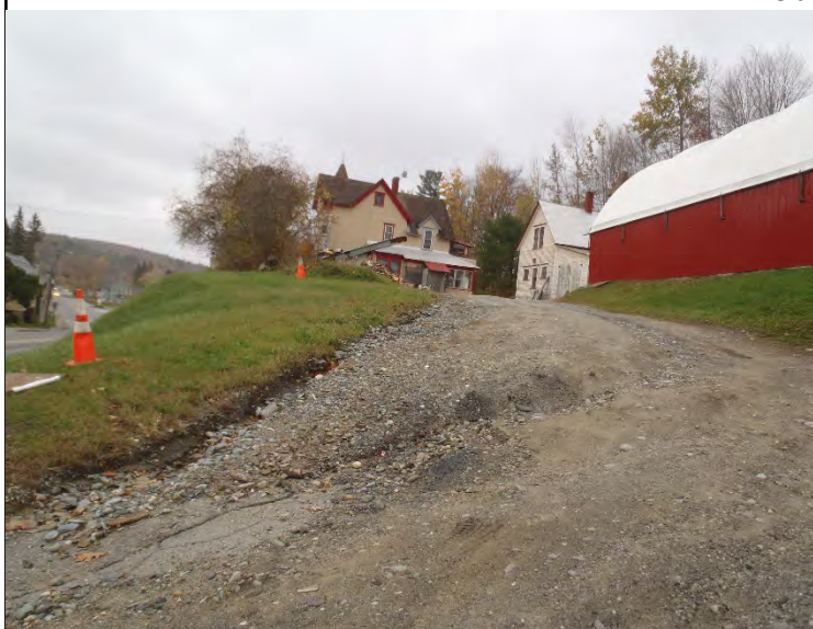
Photo 1. Driveway erosion at the home on the south corner of Hillside Street and Wolcott Street
