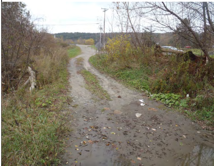
Photo 1. Sediment transport from VT Route 15 onto Wright Farm Road
