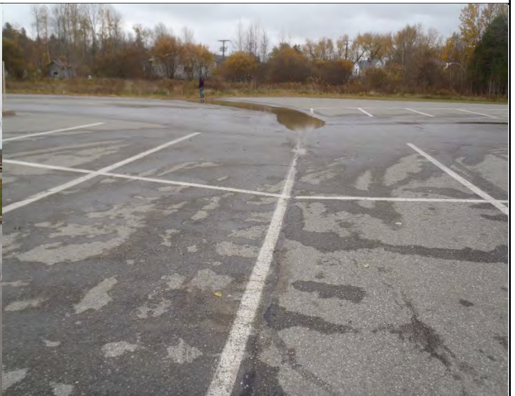
Photo 2. Parking lot drainage pattern with ponding water and potential stormwater practice location
