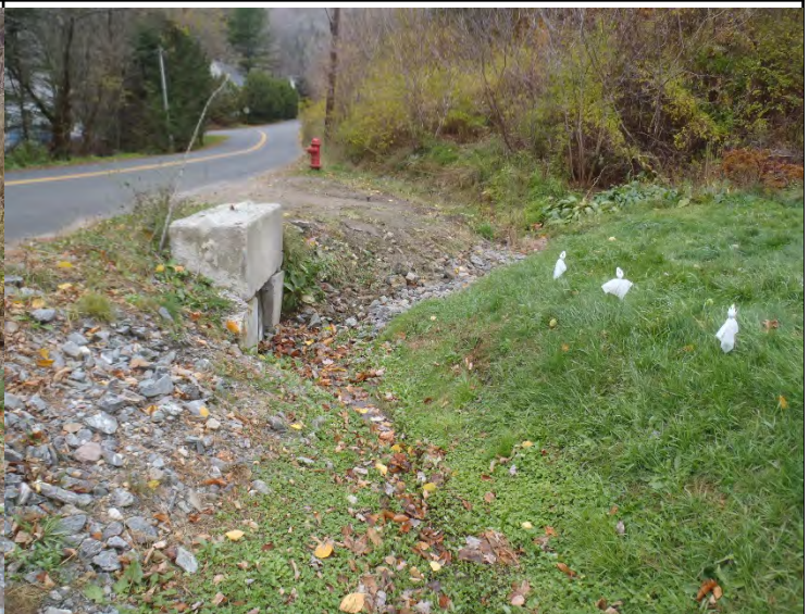
Photo 2. Slumping fire hydrant access and concrete headwall
