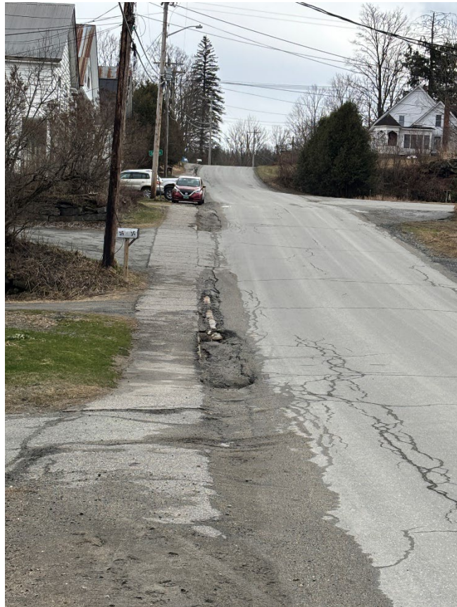
Image 2-1: Main Street Exposed Storm Drain
