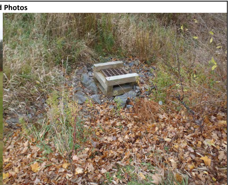
Photo 2. Existing detention basin outlet structure
