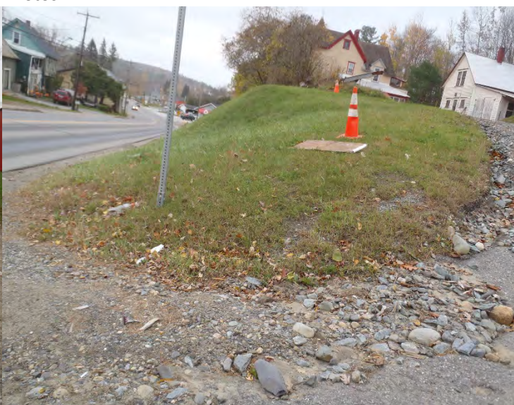
Photo 2. Sediment transport, deposition, and erosion at the intersection of Hillside Street and Wolcott Street
