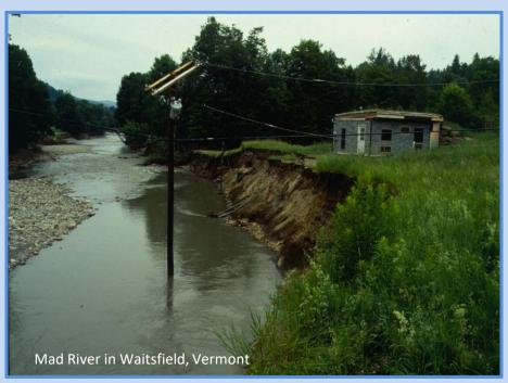
100 feet from NFIP Floodway and 8 feet above the 100yr. flood elevation.
