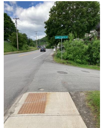
After Lower Cherry Street, the west sidewalk of South Main Street is nonexistent.
