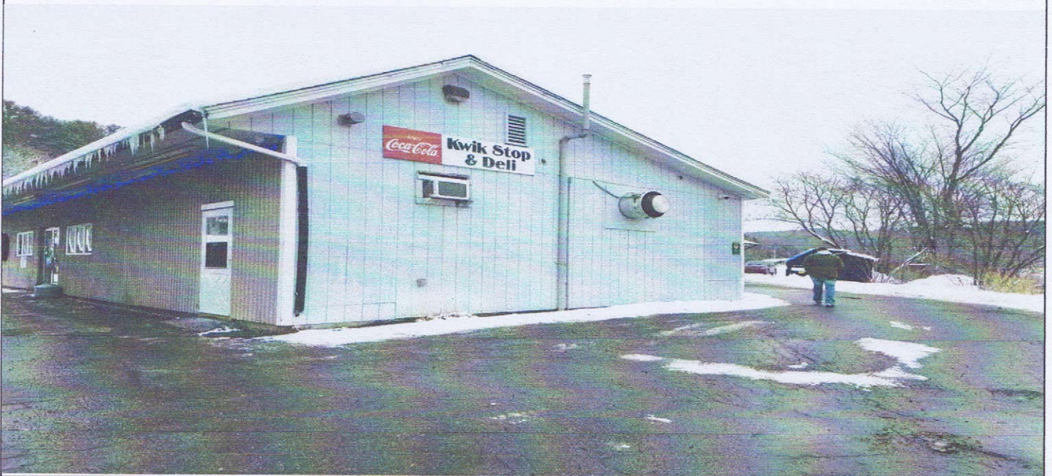
Photo Four Caption: North side taken 12/13/2025
