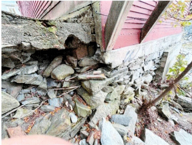
STONE WALL EROSION
