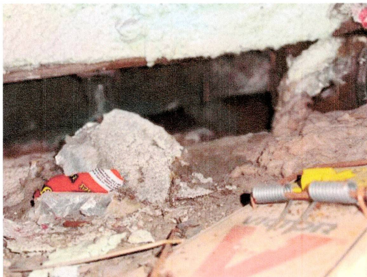
VOID UNDER EAST FOUNDATION
