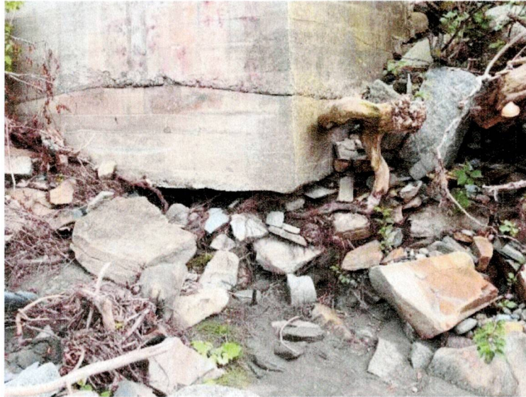
UNDERMINING AT CORNER OF FOUNDATION
