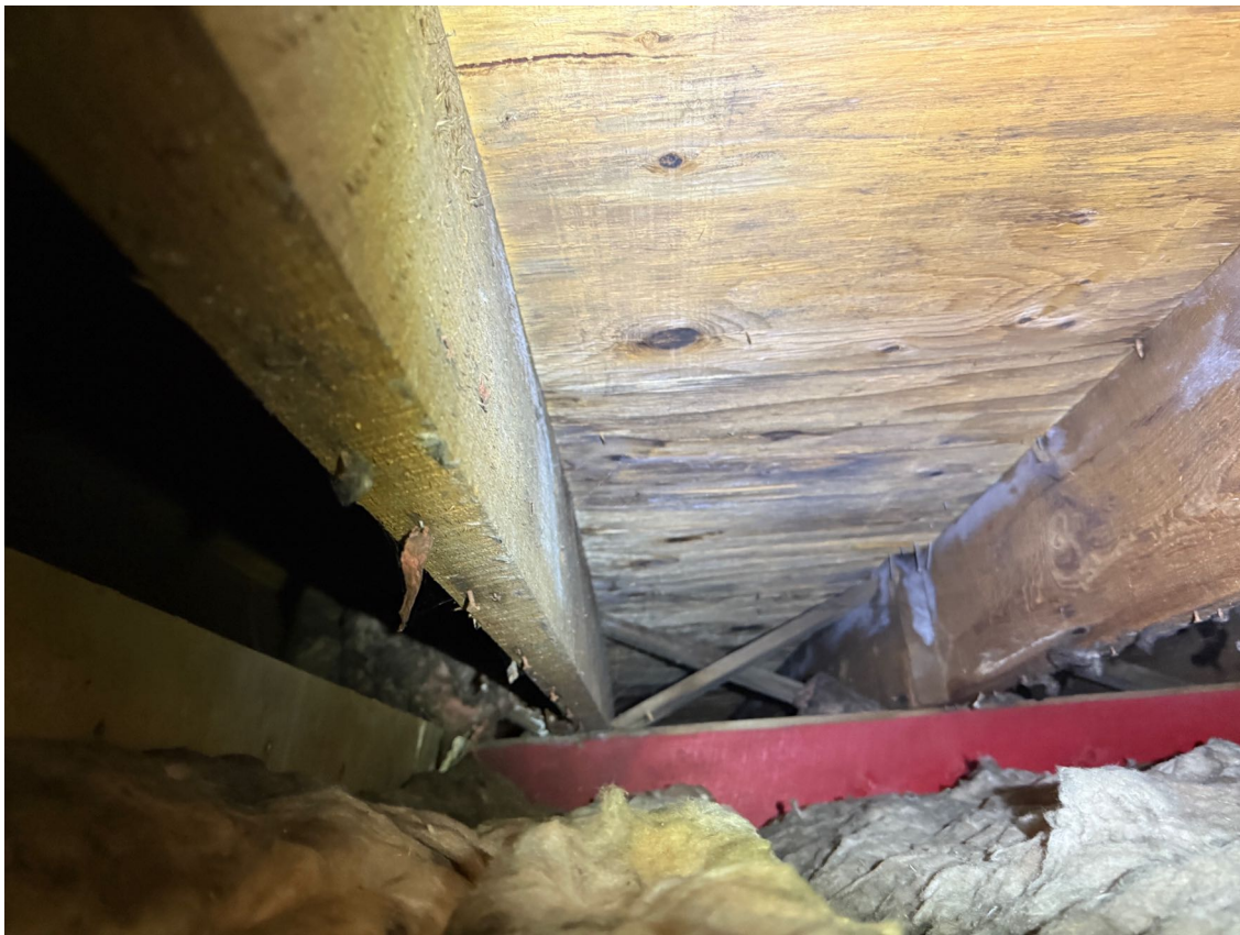
Figure 3: Existing Roof Framing
