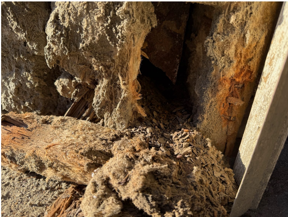
Figure 7: Steel Corrosion and Debris Accumulation at Base of Steel Column at Overhead Door
