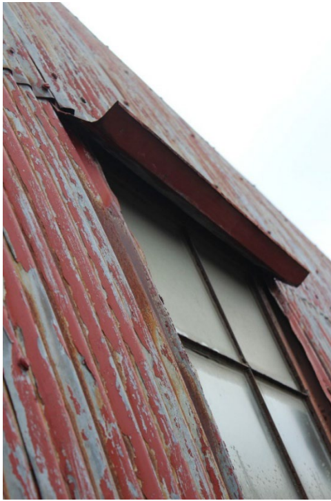
Photos 13 and 14. View NE showing the sheet metal window header and sill flashing. The header flashing is tucked under the corrugated sheet metal and has been formed to provide a narrow shade above the windows. The sill flashing protects the wooden sills. The fenestration pattern is enhanced by the juxtaposition of the flat window units and the arch shape of the south elevation.
