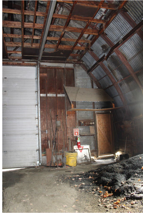
Photos 23 and 24. View east showing the added wooden stud walls north of the existing bulkhead opening (left) and south of the opening. The metal stud walls that flank the original opening each contain two structural bays. The wooden studs are butted up against the interior metal studs. The tracks for the overhead garage door are mounted to the underside of the suspended wooden frame.
