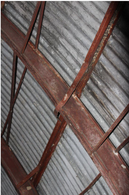
Photo 34 and 35. Detail of the intersection of a 6" I-section rib and a 2 and 5/16" I-section purlin. The ribs and purlins are made of 2 channels that are welded together back to back. The joint between the 2 channels creates a very clear groove in the middle of each flange that runs the length of the member. Each purlin/rib connection is stabilized by two pieces of 1" plate steel, each of which is nailed into the groove between the 2 channels in the I-section purlin and into the groove between the 2 channels of the I-section rib.
