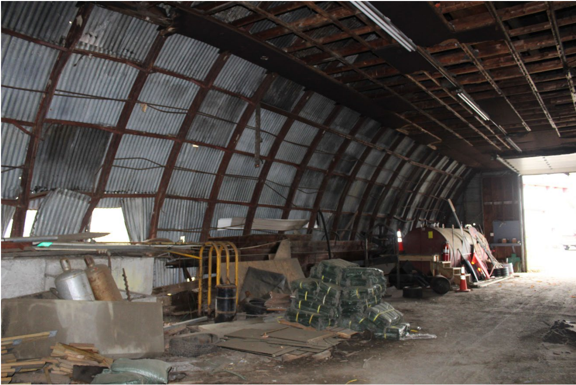
Photo 21. View NE showing the eastern portion of the north elevation and the east bulkhead. The added wood frame is supported on the header above the existing east bulkhead opening and on the header of the now infilled west bulkhead door. The large tank in the NE corner of the Quonset Gut contains gasoline.
