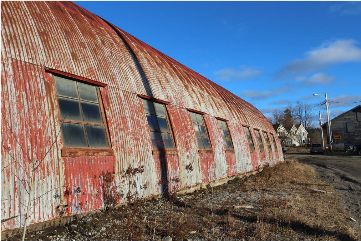
Photo 10. View NE, showing the eight, 3'-1" x 4"-7" window openings in the south elevation. The openings are spaced so that four are centered in each half of the elevation. There are two solid structural bays in the center and at each end of the elevation and single bays between each window opening. Note the short poured concrete foundation wall. The depth of the wall is unknown
