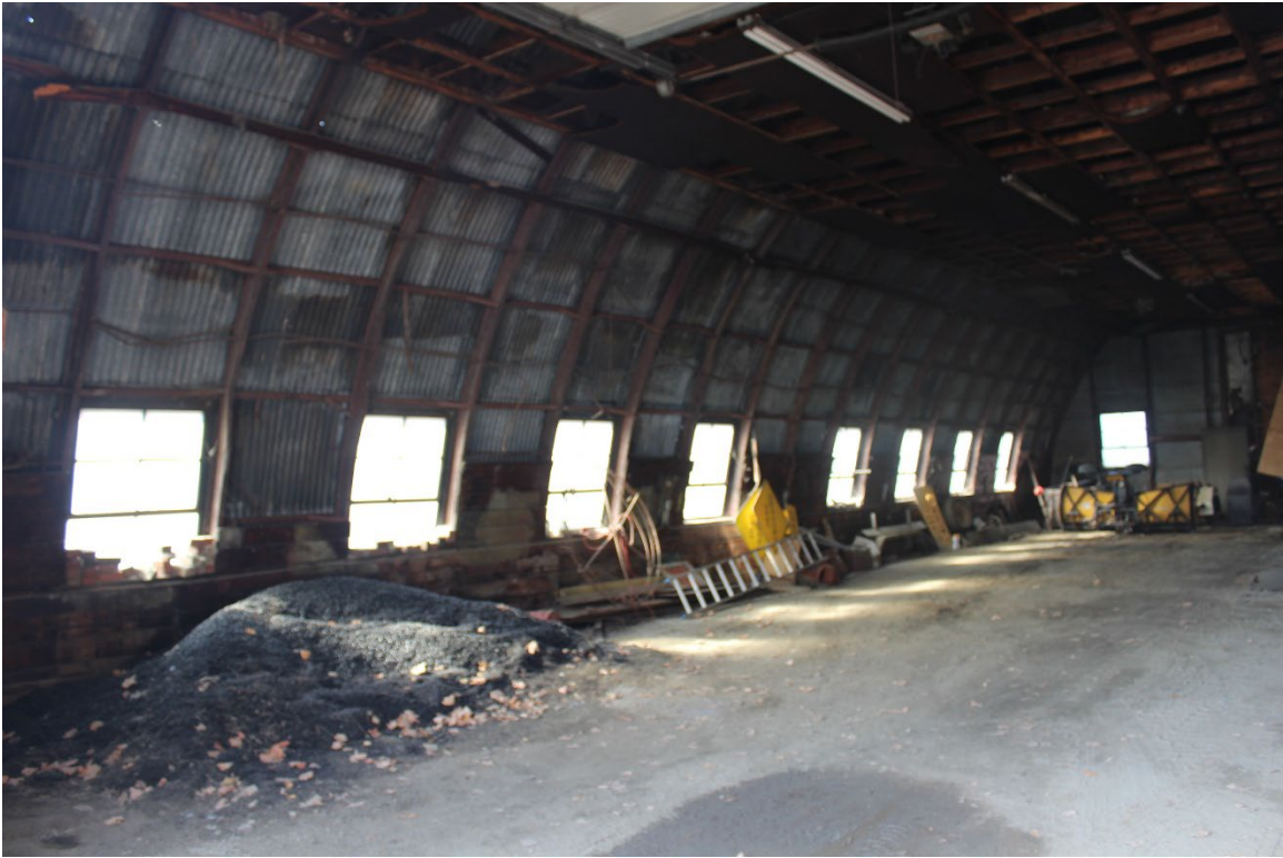
Photo 19. View SW, showing the south elevation, steel arch rib framing and the 8 windows. The windows are located so that four are centered in each half of the elevation. There are two solid structural bays in the center and at each end of the elevation and single bays between each window opening. The floor is dirt. Various materials and supplies are stored near or against the bottom of the wall.
