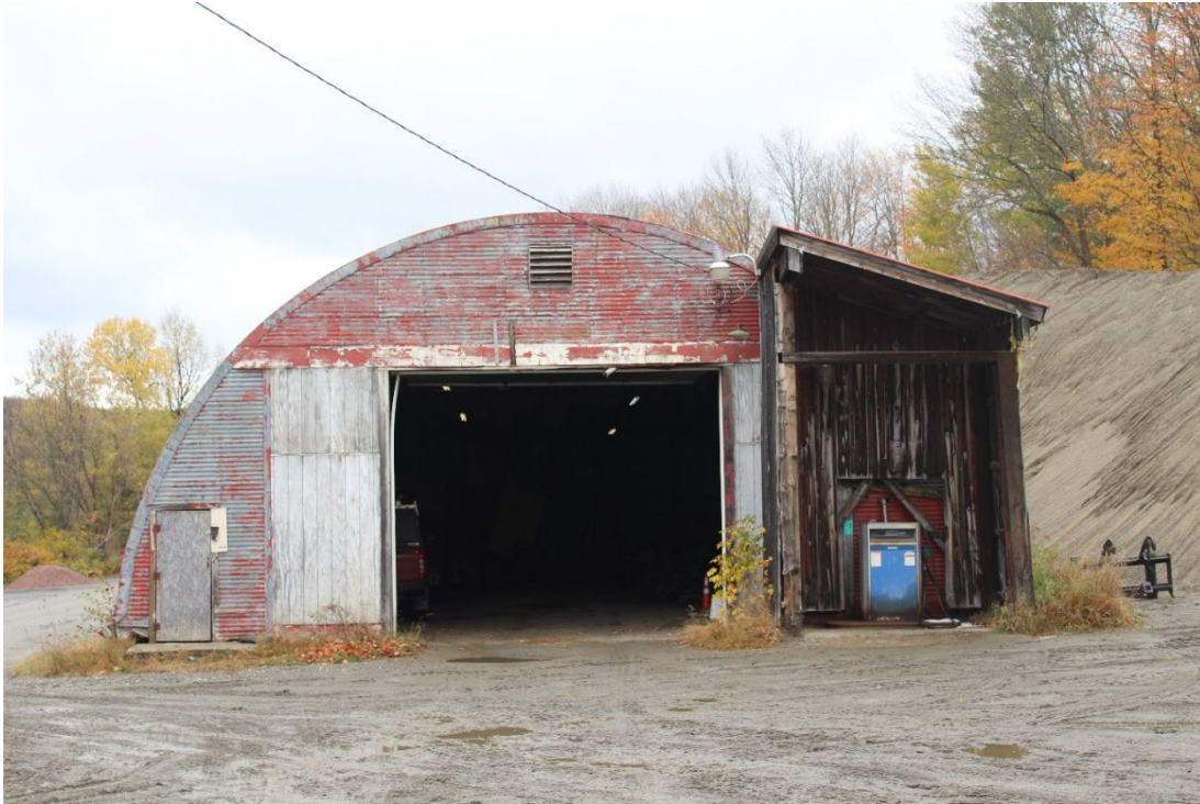
Photo 5. View W, showing the east bulkhead. Wooden stud walls sided with vertical boarding were constructed to reduce the width of the original opening. The originally opening included a wall-mounted track which extended out beyond the 40' width of the elevation and supported 4 sliding wooden doors. The doors and track were removed when opening was altered. Sheet metal flashing that now overs the track area is tucked under the historic crimped flashing.
