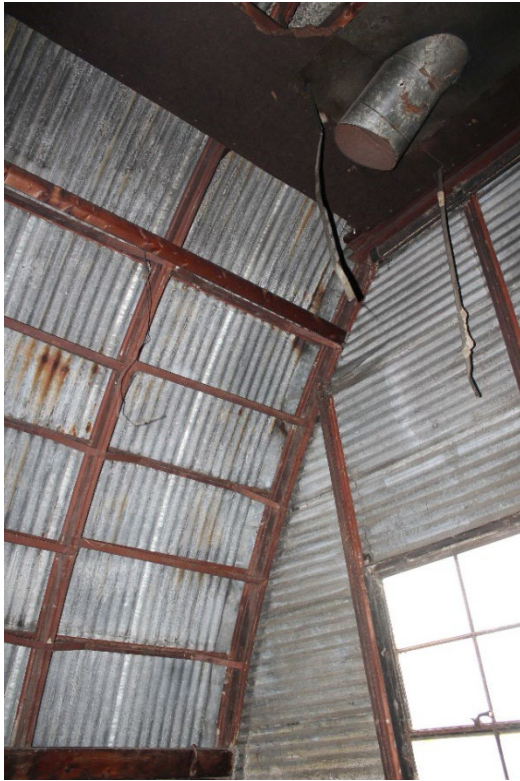
Photo 29, left, view SW showing the junction of the south arch rib framing and the west stud wall framing. The I-section studs are smaller than the I-section ribs. The added boarding that carries the electrical conduit is adjacent to the purlin immediately below the added wood frame. Photo 30, right. The added wood frame makes it difficult to see the ribs and purlins above. The suspended frame is supported along its length by 2 x 4s that are nailed to the wood frame and to each steel rib above
