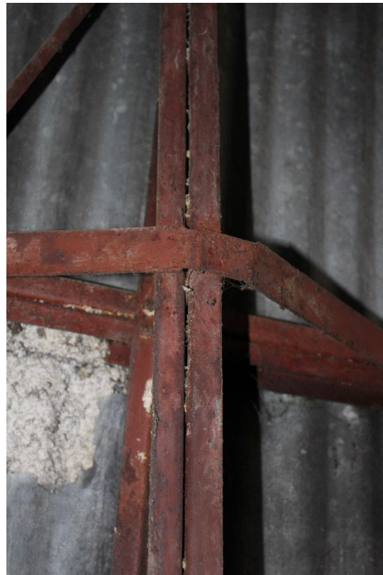
Photo 34 and 35. Detail of the intersection of a 6" I-section rib and a 2 and 5/16" I-section purlin. The ribs and purlins are made of 2 channels that are welded together back to back. The joint between the 2 channels creates a very clear groove in the middle of each flange that runs the length of the member. Each purlin/rib connection is stabilized by two pieces of 1" plate steel, each of which is nailed into the groove between the 2 channels in the I-section purlin and into the groove between the 2 channels of the I-section rib.
