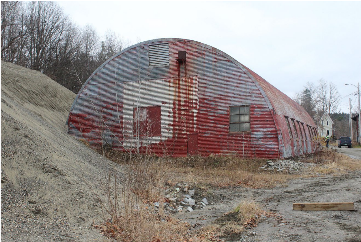
Photo 4. View NE, showing the west bulkhead and the south elevation. The original wide opening in the west bulkhead has been infilled with sheet metal. The single window in the south corner matches the windows on the south elevation but is located higher in the wall. The louver at the top of the wall is larger than the east bulkhead louver and may be original because it matches a louver style shown in several Quonset Hut Manuals (US Navy Seabees Museum). Note the close proximity of the sandpile to the Quonset Hut.
