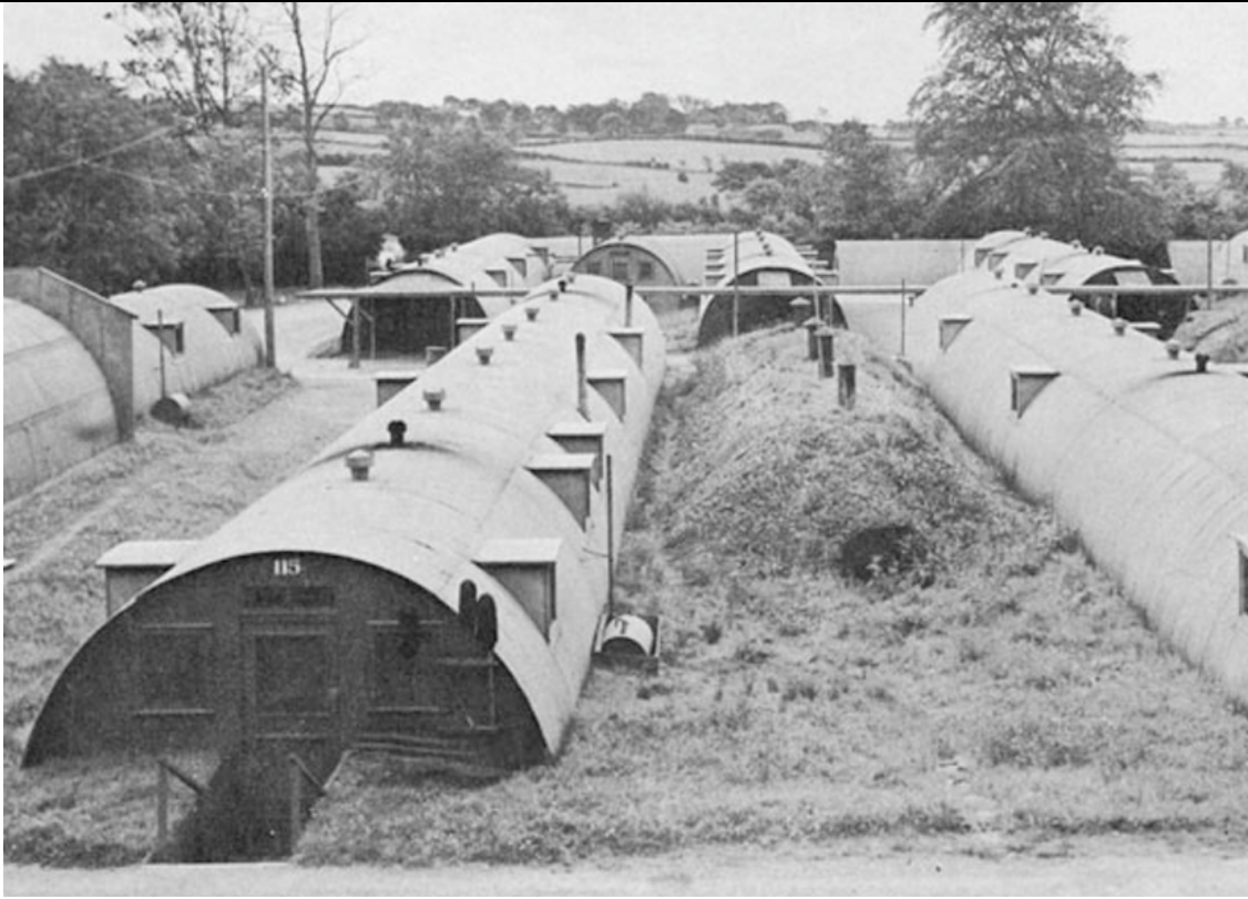
Photo from the website U.S. Navy Quonset Hut, Weapons of Mass Construction . Several of the Utility Buildings in the second row of the photo appear to have very wide bulkhead openings.
