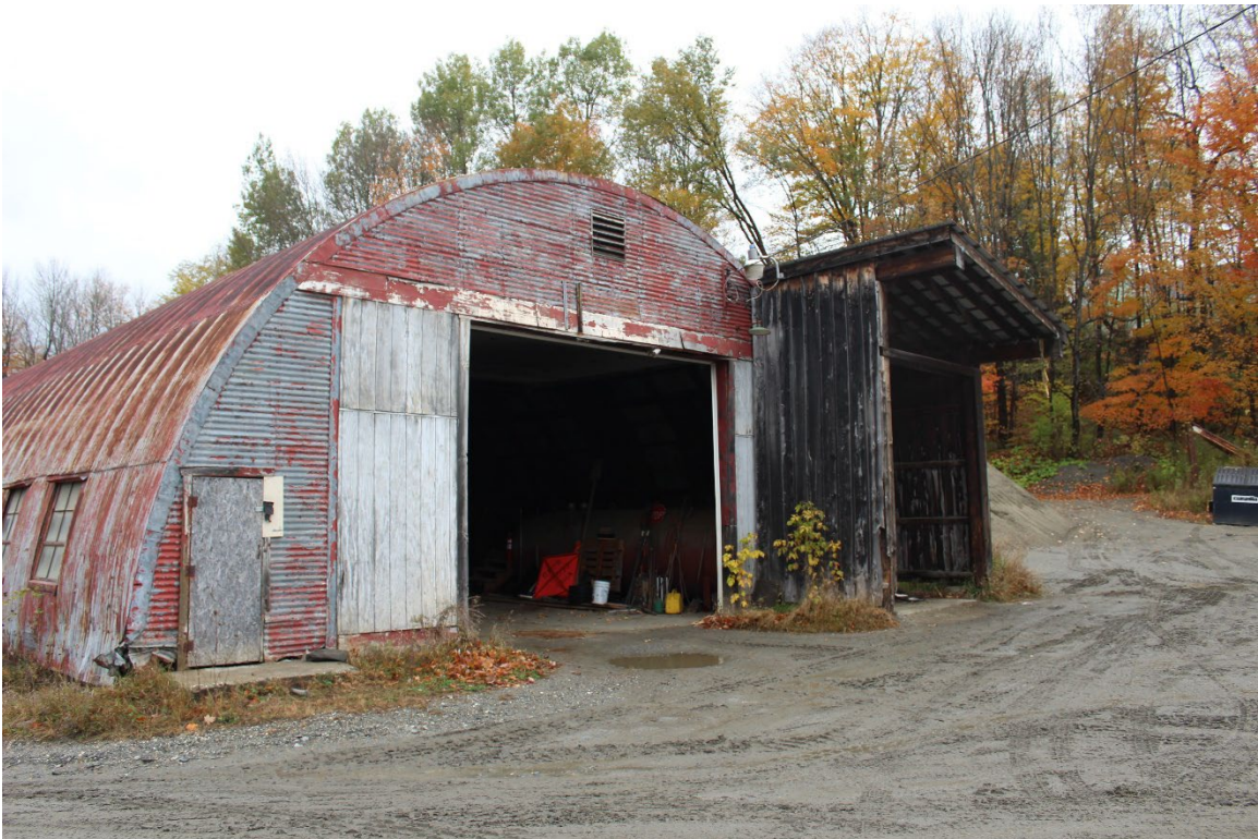
Photo 2. New NW, showing the east bulkhead. The centered garage bay opening is flanked by narrow sections of wall sided with vertical boarding rather than horizontally-oriented corrugated metal. The man door in the south corner of the bulkhead is made of single piece of fiberboard. The non-historic shed-roofed structure north of the garage bay door covers the Town Garage gasoline pump and is not structurally attached to the Quonset Hut.
