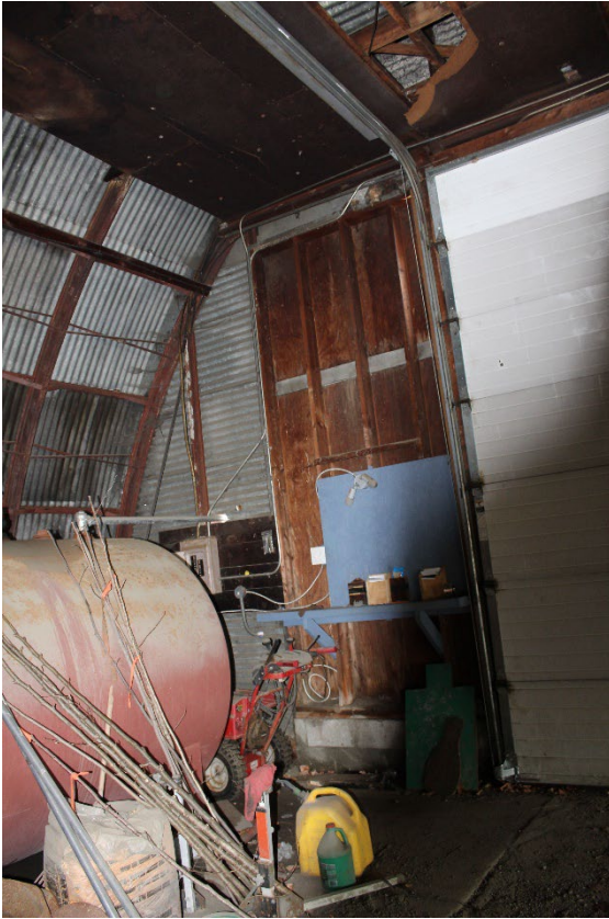
Photos 23 and 24. View east showing the added wooden stud walls north of the existing bulkhead opening (left) and south of the opening. The metal stud walls that flank the original opening each contain two structural bays. The wooden studs are butted up against the interior metal studs. The tracks for the overhead garage door are mounted to the underside of the suspended wooden frame.
