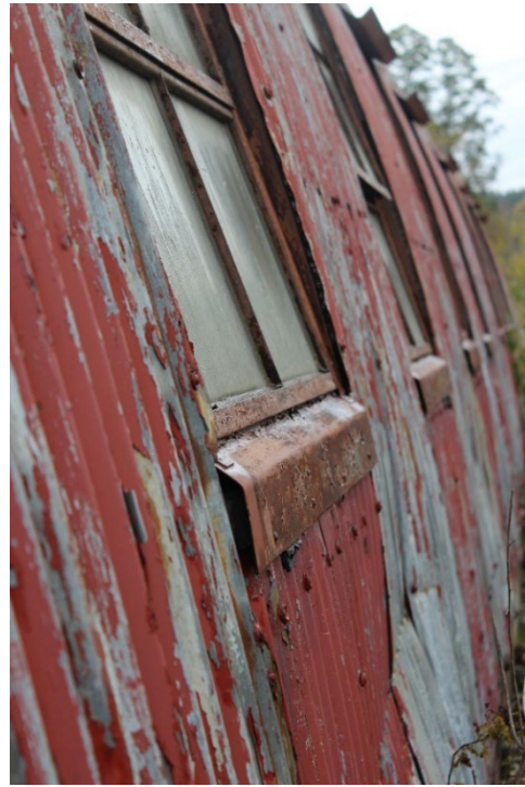
Photos 13 and 14. View NE showing the sheet metal window header and sill flashing. The header flashing is tucked under the corrugated sheet metal and has been formed to provide a narrow shade above the windows. The sill flashing protects the wooden sills. The fenestration pattern is enhanced by the juxtaposition of the flat window units and the arch shape of the south elevation.
