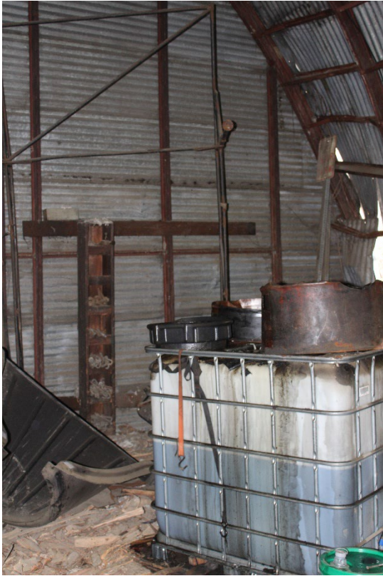
Photo 26, left. View NW showing the stud wall north of the former west bulkhead door. The I-section wall studs are slightly smaller than the I-section arch ribs. Photo 27, right. View SW, showing a damaged I-section Stud in the west bulkhead. The I-section ribs, purlins and studs are made of 2 channels joined back to back. Note the groove or joint in the center of the flange on the I-section stud.
