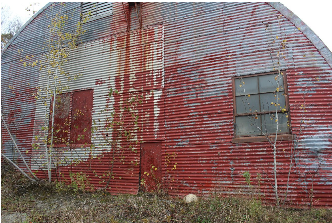
Photo 15. View NE, west bulkhead. The now infilled wide, centered opening appears to have been the same height as the opening in the east bulkhead. The added paired window openings in the patched area are taller and narrower than the original windows; the sill flashing has been retained but is narrower than the sill flashing associated with the original windows.
