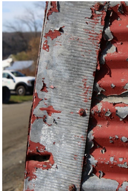
PPHotos 6 and 7. View west, showing the crimped end wall flashing at the southeast building corner. The end wall flashing extends around the perimeter of the east and west bulkhead elevations and is tucked beneath the corrugated metal sheathing on the north and south elevations.
