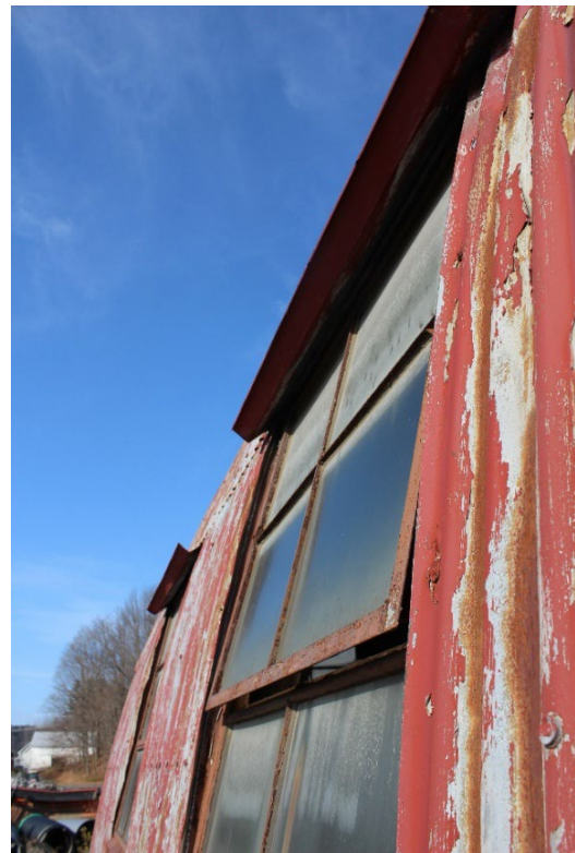
Photos 11 and 12. View west showing a typical four-light over-two light metal window. The four-light top windows are side-hinged to operate as louvers. The bottom two-light windows are fixed. The individual lights are horizontally-oriented. The flat window units are mounted into the arch-shaped south elevation.
