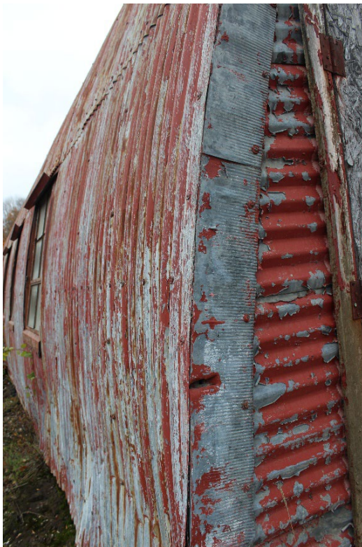
PPHotos 6 and 7. View west, showing the crimped end wall flashing at the southeast building corner. The end wall flashing extends around the perimeter of the east and west bulkhead elevations and is tucked beneath the corrugated metal sheathing on the north and south elevations.
