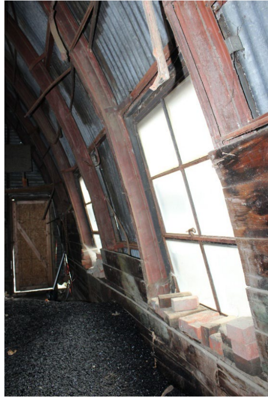
Photo 40. View west (left) and Photo 41. View east. The four-light upper windows are side-hinged to open as louvers. The bottom two-light windows are fixed. Each flat window unit spans the width of a structural bay. Each bay is defined by 2 of the 21 steel arch ribs. Window sills are wooden.
