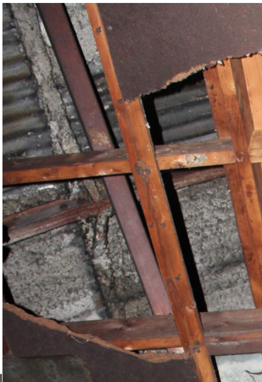
Photo 31, left, view SW. A splice plate that joins 2 sections of an arch rib is visible on the left side of the photo, just below the north/south oriented framing member. Photo 32, right, view east. A splice plate in the third furthest rib is barely visible above the wood frame.
