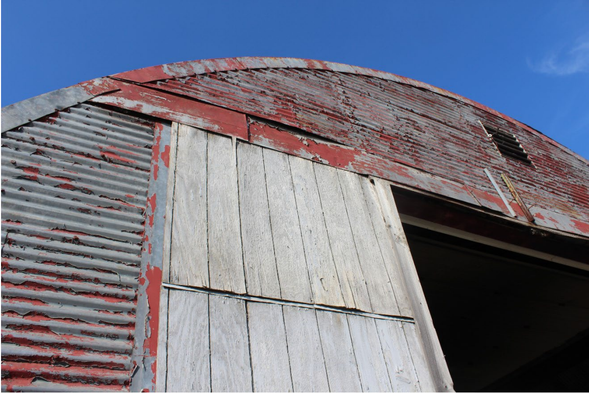
Photo 8. View W. The wall mounted track that held the 4 original sliding wooden garage doors was removed. Wide flashing was installed over the area of track attachment. The added flashing is tucked under the historic crimped flashing the overs the joint between the bulkhead and the arched rib framing.
