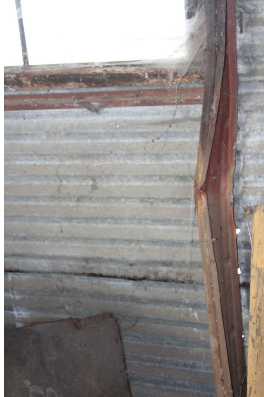
Photo 26, left. View NW showing the stud wall north of the former west bulkhead door. The I-section wall studs are slightly smaller than the I-section arch ribs. Photo 27, right. View SW, showing a damaged I-section Stud in the west bulkhead. The I-section ribs, purlins and studs are made of 2 channels joined back to back. Note the groove or joint in the center of the flange on the I-section stud.
