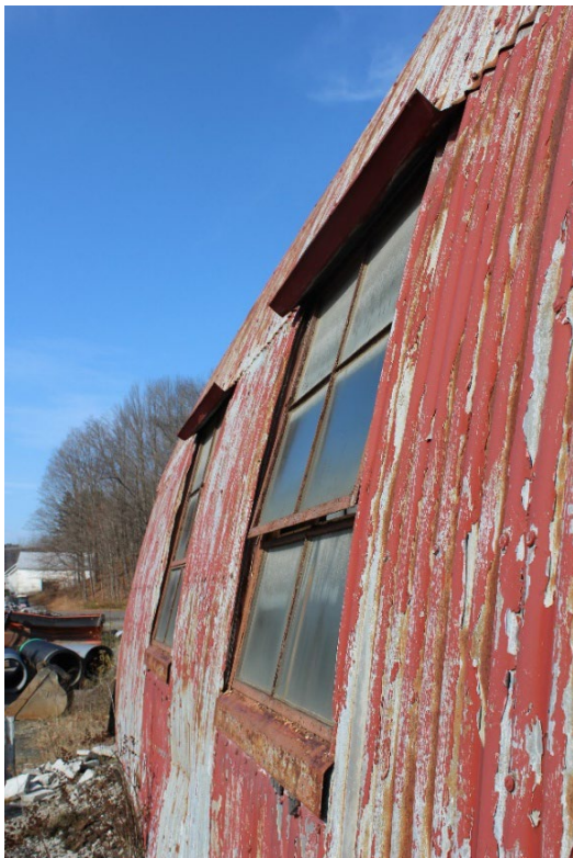
Photos 11 and 12. View west showing a typical four-light over-two light metal window. The four-light top windows are side-hinged to operate as louvers. The bottom two-light windows are fixed. The individual lights are horizontally-oriented. The flat window units are mounted into the arch-shaped south elevation.
