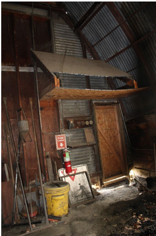
Photos 38, left. View SE showing the electrical breaker box on the east bulkhead wall. Conduit runs from the box up along the metal stud to the right of the box. Photo 39, right, showing a lighting fixture mounted on the boarding that carries the conduit.
