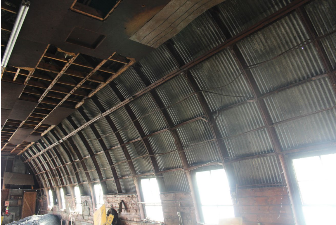
Photo 33. View SE. The steel arch rib framing consists of twenty-one 6", I-section ribs spaced 4' on center that enclose 20 structural bays. Each rib is apparently assembled from three spliced sections. The arch frame also includes 2- 5/16" I-section purlins which run horizontally for the length of the building and are screwed to the outside or top flange of the ribs. The frame also incorporates standard cross bridging which is centered between the purlins and provides lateral stability.
