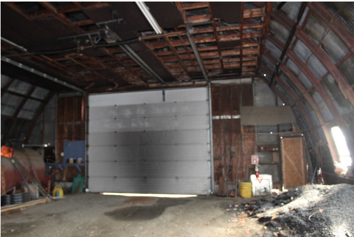
Photo 22. View NE showing the interior of the east bulkhead. The width of the original opening was reduced by the construction of wood stud walls inboard of the historic metal stud framing. The added man door was let into the metal stud-framed SE corner. . Note that the added suspended wood frame spans the width of the original opening.
