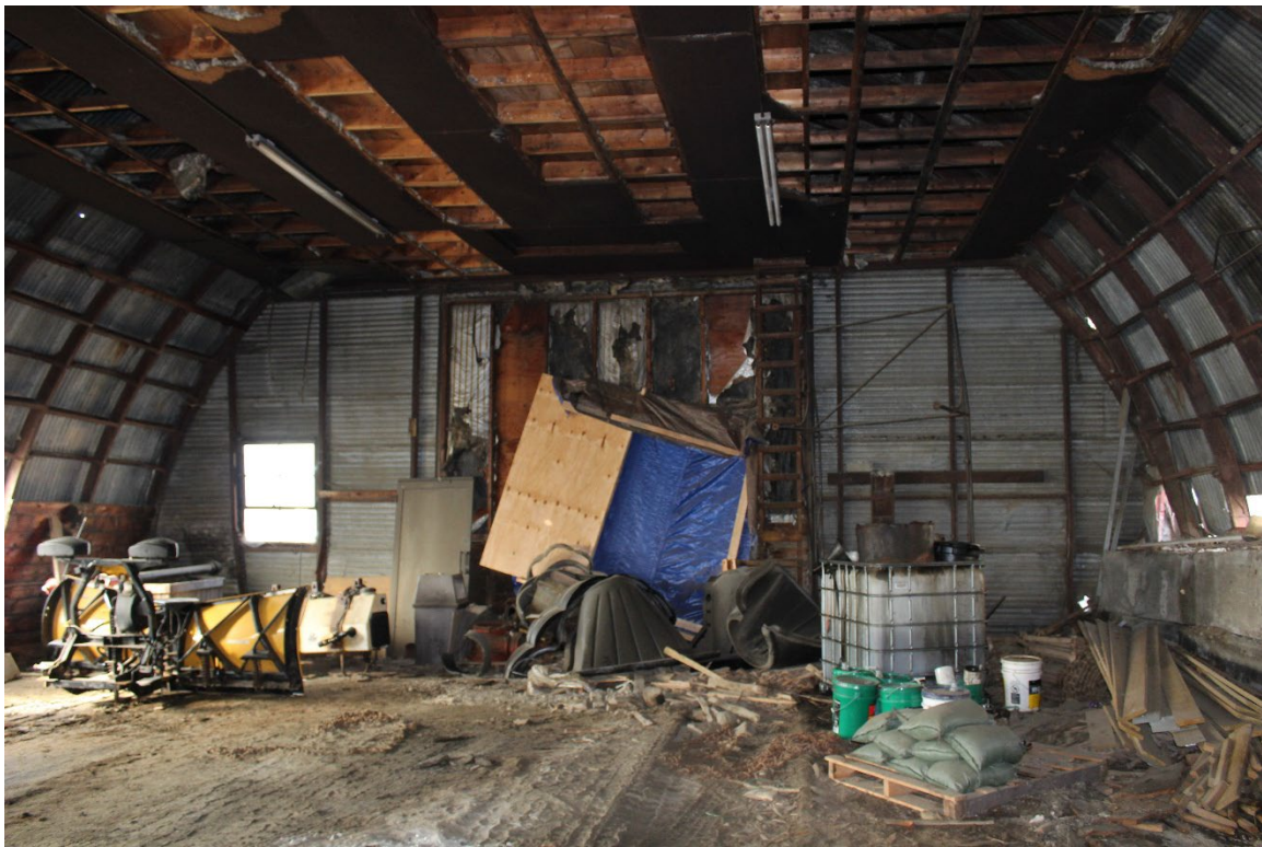
Photo 25. View W, showing the west bulkhead. The wide opening has been infilled but its original width does not appear to have been altered. The metal stud walls that flank the opening are each four bays wide. The stud bays immediately adjacent to the original opening are significantly narrower than the other bays.
