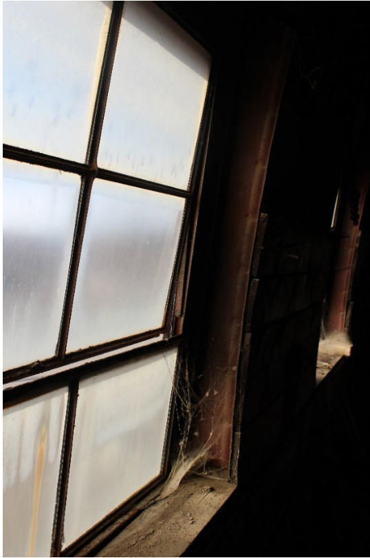
Photo 40. View west (left) and Photo 41. View east. The four-light upper windows are side-hinged to open as louvers. The bottom two-light windows are fixed. Each flat window unit spans the width of a structural bay. Each bay is defined by 2 of the 21 steel arch ribs. Window sills are wooden.
