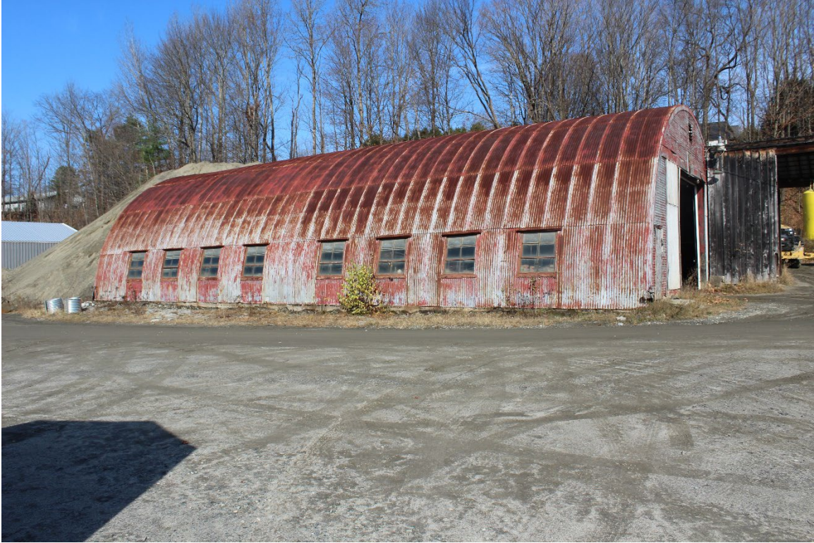
Photo 1. Hardwick Quonset Hut/Hardwick Town Garage. View NW, showing the south and east bulkhead elevations. Available architectural plans for a Quonset Hut refer to the vertical, end elevations as bulkheads. The 8 windows in the south elevation are grouped so that 4 are centered in each half of the elevation.
