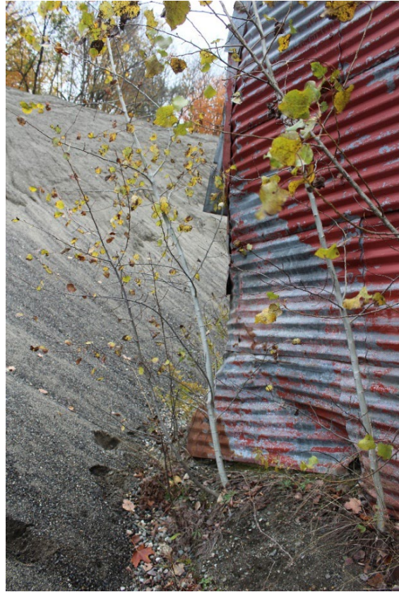
Photos 16 and 17. View NE, showing damage to the SW (left) and NW corners of the west bulkhead. Note the crimped end wall flashing around the perimeter of the west bulkhead.
