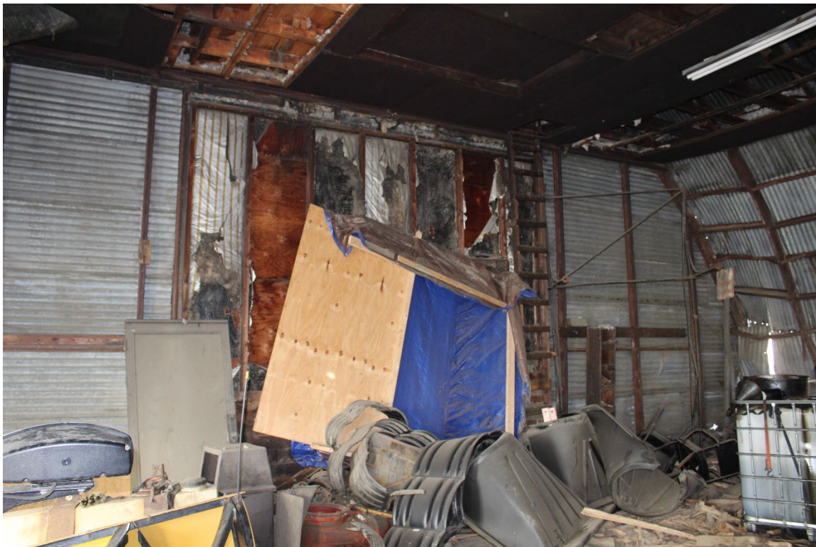
Photo 28. View NW. The stud walls on both sides of the former opening in the west bulkhead are each four bays wide; the interior bays that flank the opening are quite narrow. A wooden frame has been added within the original opening. The wood posts are attached directly to the metal studs that framed the opening. The wood header is several inches below the original channel plate. The wood frame may have been added to provide a nailing surface when the west opening was infilled.
