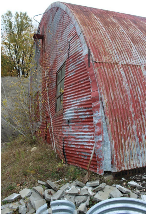
Photos 16 and 17. View NE, showing damage to the SW (left) and NW corners of the west bulkhead. Note the crimped end wall flashing around the perimeter of the west bulkhead.
