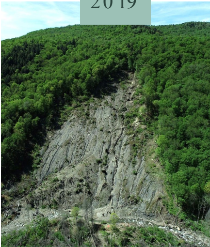
Cotton Brook Landslide, Waterbury, VT
