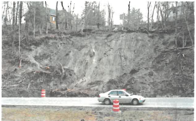
Glenside landslide site on April 22, 2004, 3 days after a major slope failure occurred. Photo by George Springston.
