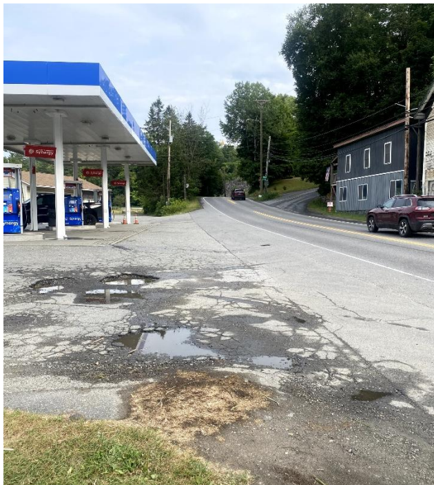
Figure 2 Study Corridor (Mill Street, EB)
