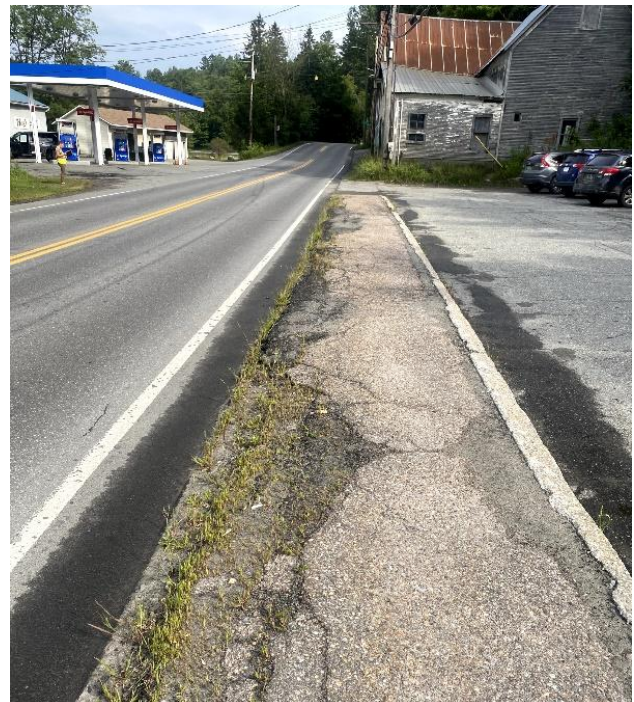
Figure 9 Existing Sidewalk (east of Sumner St.)
