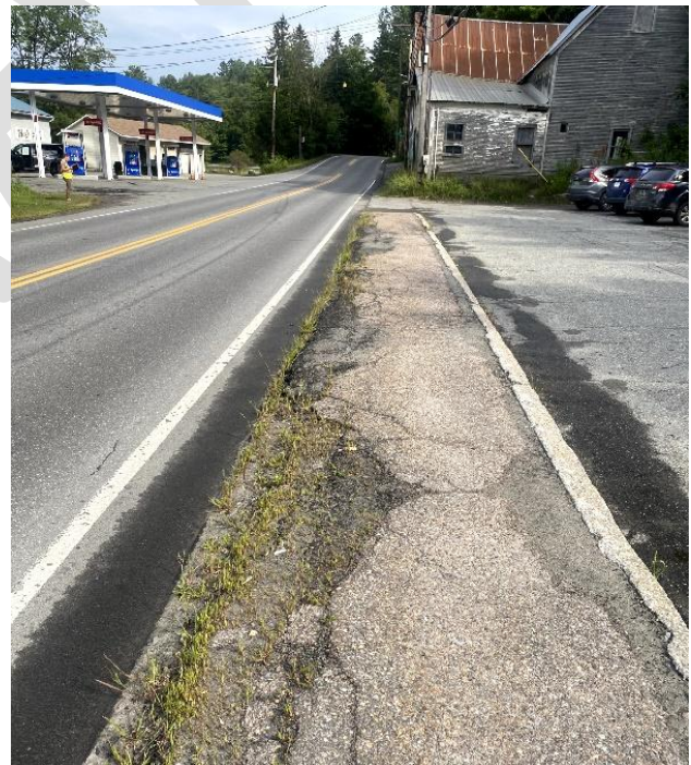
Figure 9 Existing Sidewalk (east of Sumner St.)
