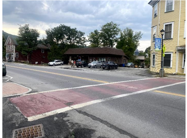
Figure 3 Study Corridor (South Main Street, SB)
