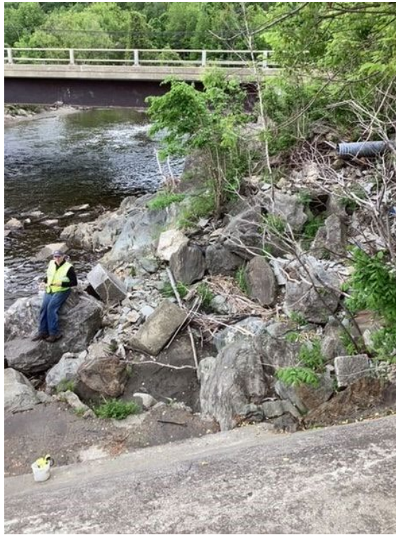
Auxiliary Spillway discharges onto a splash pad that appears to be founded on bedrock.
