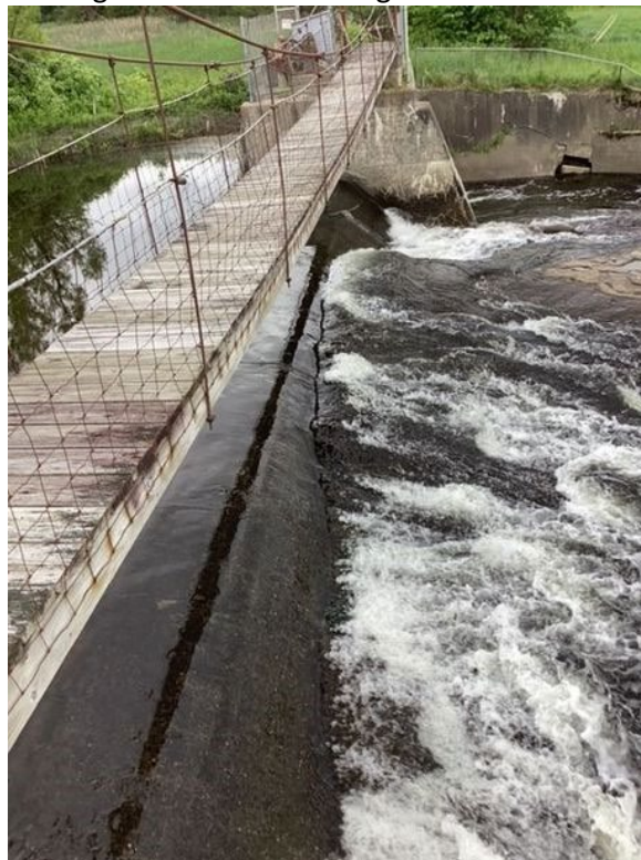
Weir section on left side.
