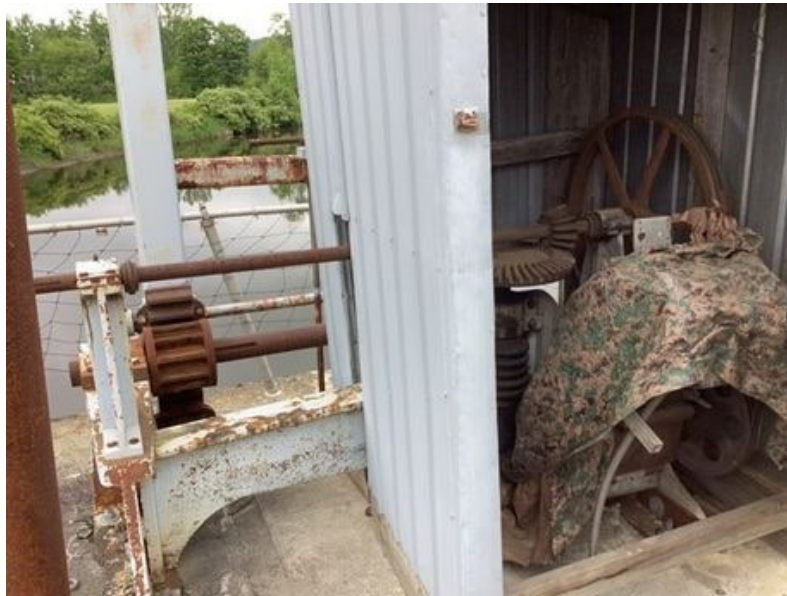
Gate across wooden spillway cable bridge.
