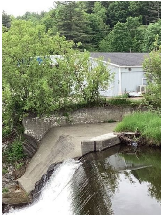
Auxiliary spillway at the right abutment.
