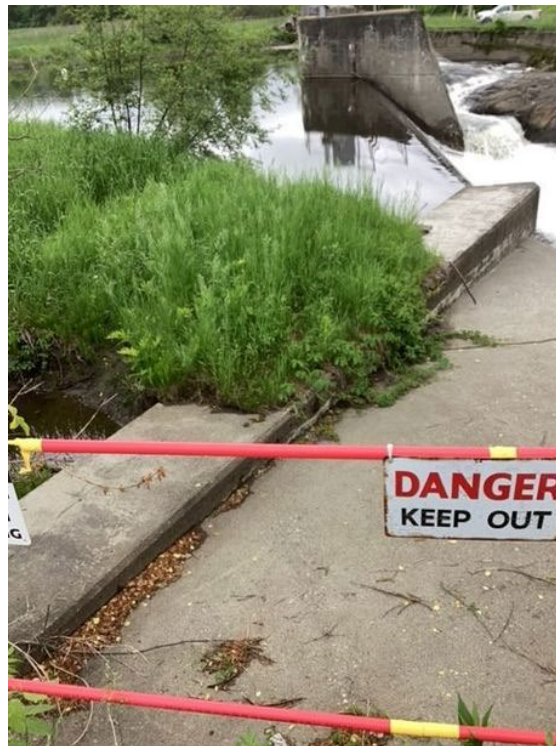
Broad crested auxiliary spillway weir from right abutment.
