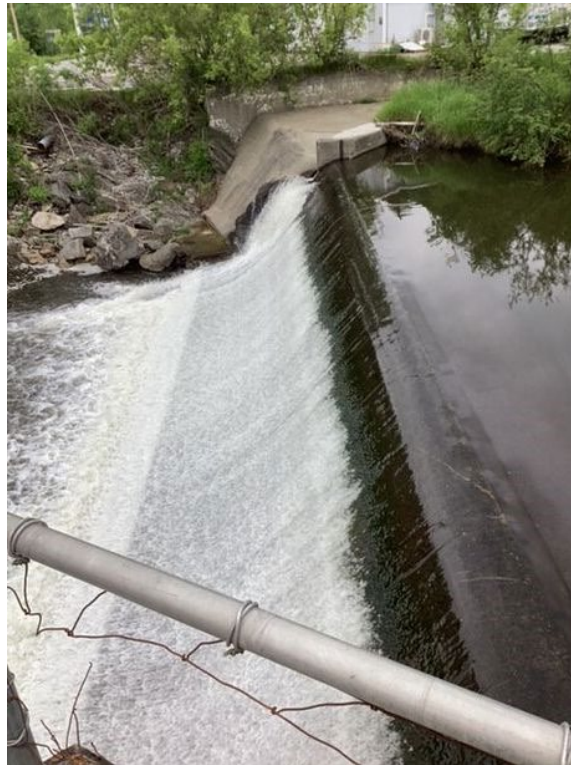
Ogee weir section on right side of dam.
