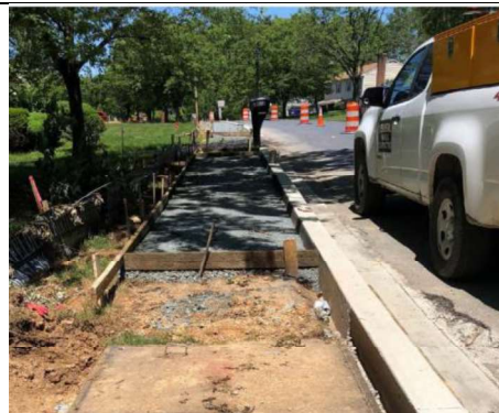
Sidewalks being replaced.
