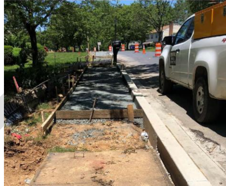
Sidewalks being replaced.
