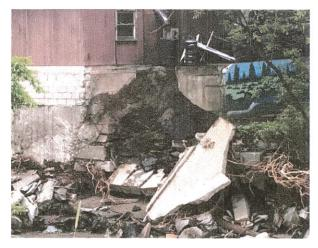
July 2024 – The foundation of Civic Standard Building was removed by flooding. Estimated cost to repair may be as much as \$100,000. Adjoining town-owned green space (Peace Park) has damaged retaining walls. No cost estimate or funding plan in place yet.
