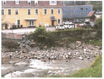
July 2023 and July 2024 – The Town's retaining wall next to the North Main Street Bridge was damaged and will need to be repaired. No cost estimate or funding source identified yet.
