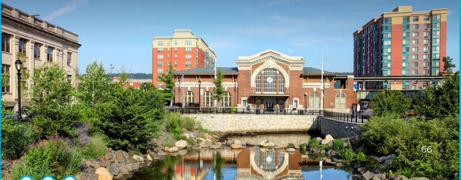
Stream daylighting of the Saw Mill River in downtown Yonkers, New York. (Source: Getty)
