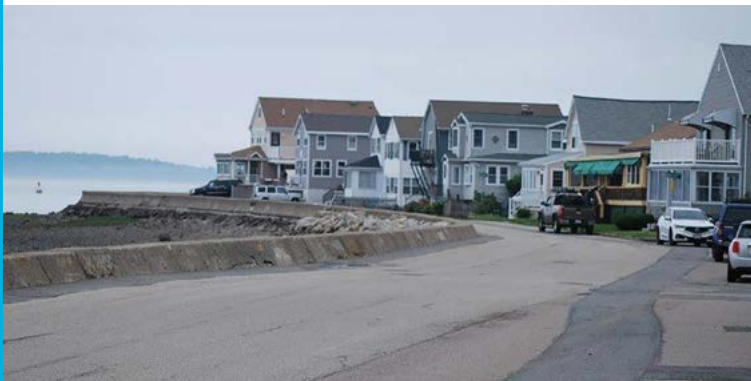
A proposed increase in the height of the Fort Point Road seawall (right) up to 2 feet above its current height (left) is being explored as a way to reduce flood risk in Weymouth. (Source: © Tighe & Bond)
