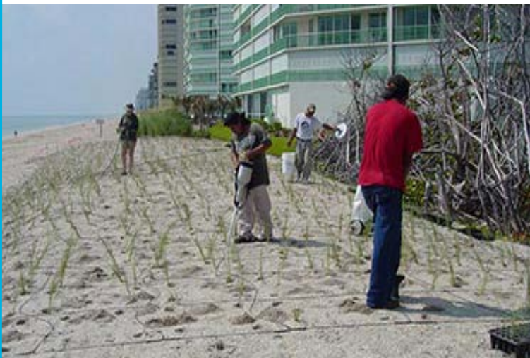
Dune grasses used to stabilize beach sand were part of a locally-funded beach and dune restoration project on South Hutchinson Island. (Source: St. Lucie County )
