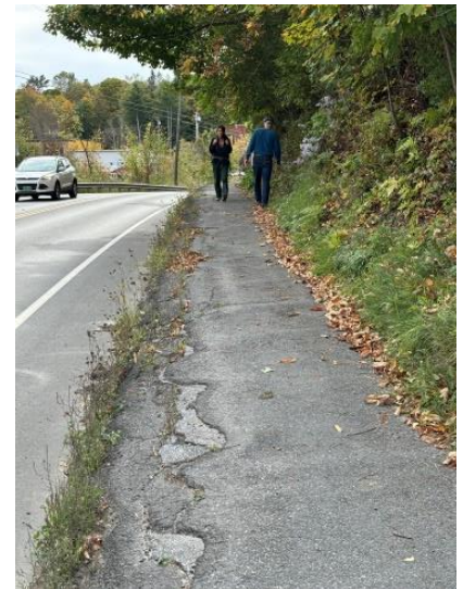
East sidewalk is not adequate in places for a wheelchair or other forms of mobility assistance.
