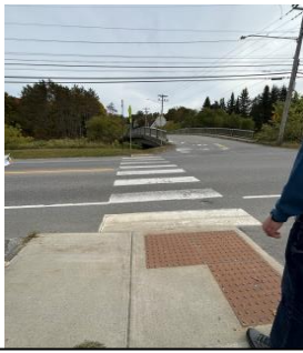
Upgraded cross walk at the Cottage Street Bridge
