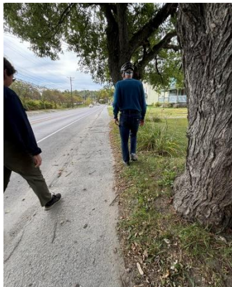
Near Granite Street – no separation from Wolcott Street
