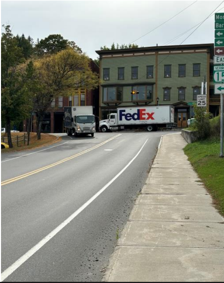
View to the 3-way Intersection from Wolcott Street – improved sidewalk and 25 mph sign for Main Street.
