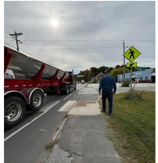
Near Cottage Street – no separation and a cracking, crumbling sidewalk.
