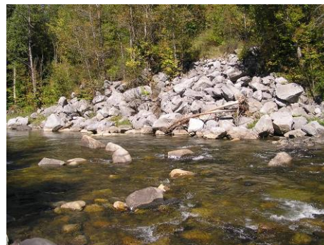
Figure 3. R26 Riprap at river’s abutment with railroad bed
