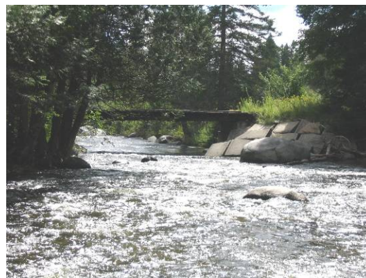
Figure 7. Problem bridge and channelization in R30B
