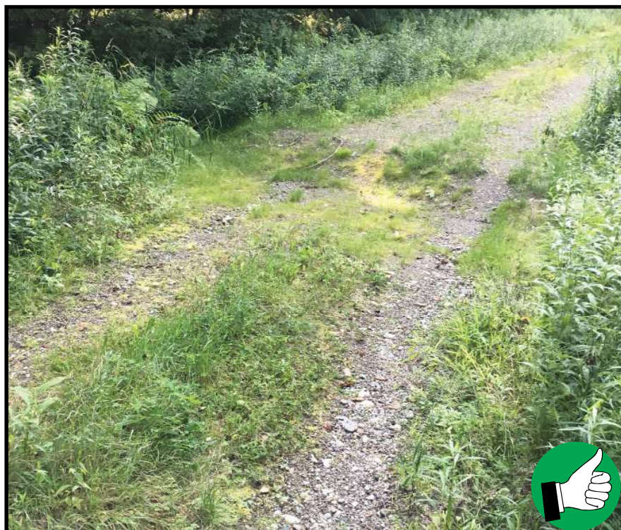
Good installation of a water bar along an access road.
