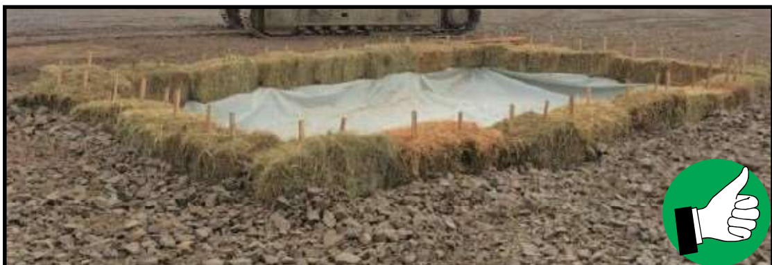
ABOVE GRADE STRAW BALE CONCRETE WASHOUT DETAIL
