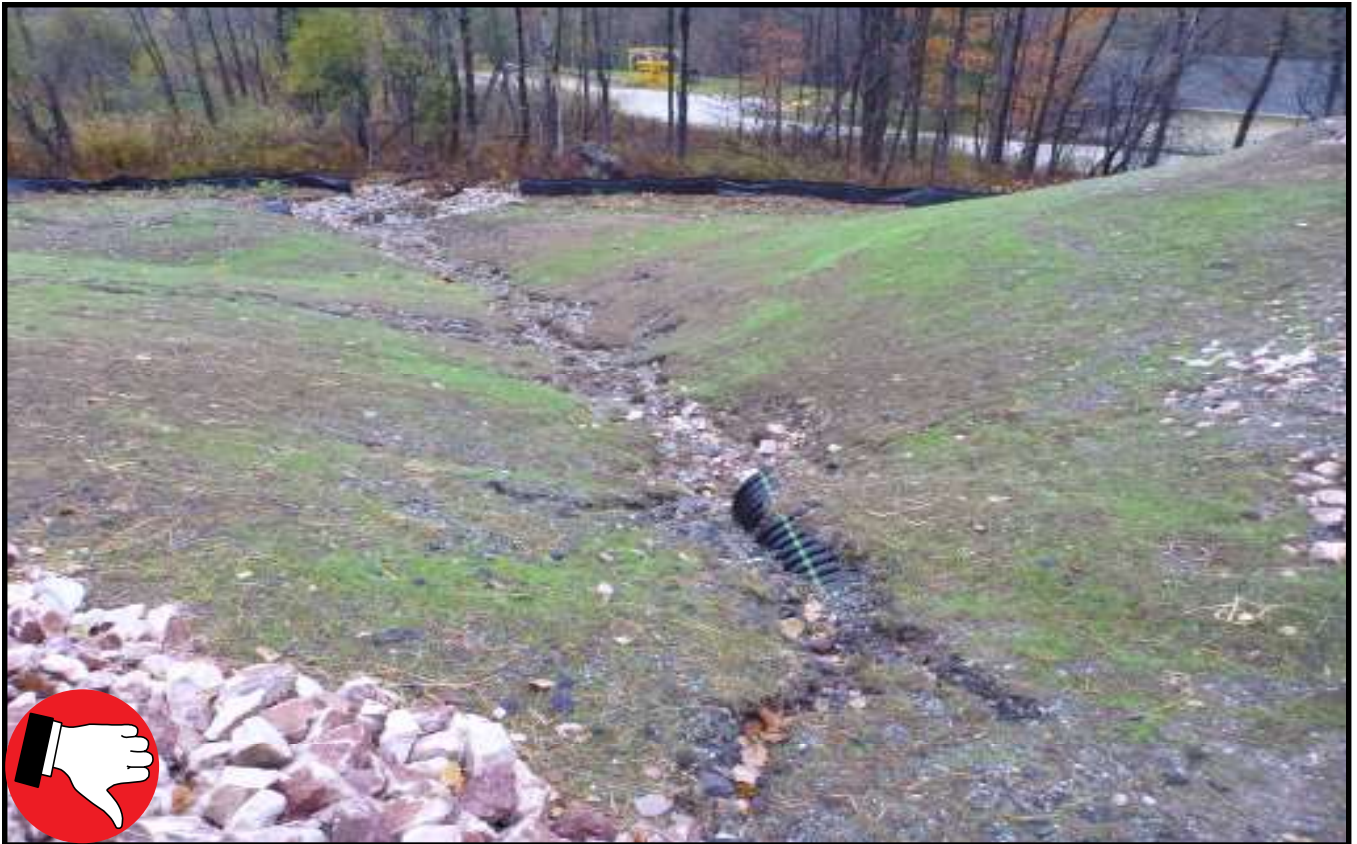
Before installing rock outlet protection
