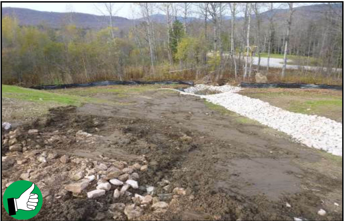
After installing rock outlet protection
