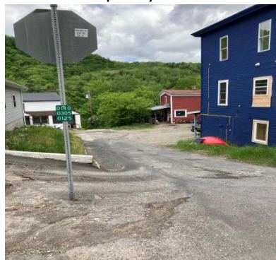
Intersection of South Main Street and Farr Street – after a minimal rain event.
