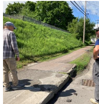
East sidewalk is not adequate in places for a wheelchair or other forms of mobility assistance.
