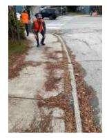
broken and storm drains are either within the actual sidewalk or have aspects which make travel difficult. The section of sidewalk near the public parking area has an asphalt patch which makes travel nearly impossible for most pedestrians and impossible for anyone who needs mobility assistance. Between the Post Office parking lot and Perry Lane Hill, there are cables set into the sidewalk which are in the pedestrian path.
