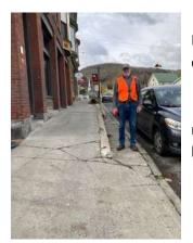
4) The east sidewalk splits into a two-level situation directly before the Holton Hill intersection. The upper level of the sidewalk has 6 ½ feet of width and then drops substantially and has an additional 2 feet.
