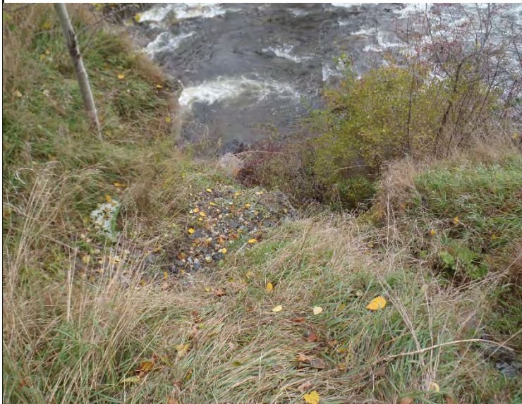
Photo 1. Marginal erosion on the northwest corner of the bridge
