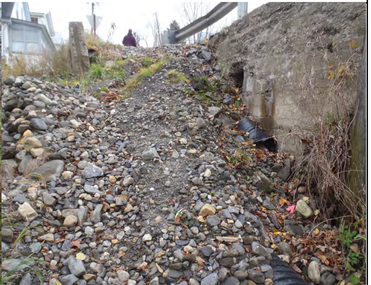
Photo 2. Substantial erosion on the southeast corner of the bridge
