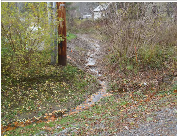
Photo 1. Destabilized open ditch lacking erosion control
