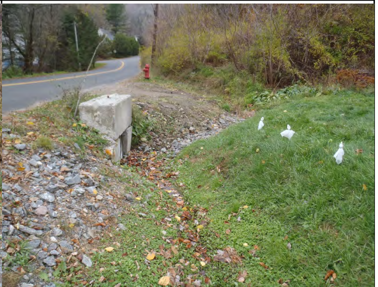
Photo 2. Slumping fire hydrant access and concrete headwall
