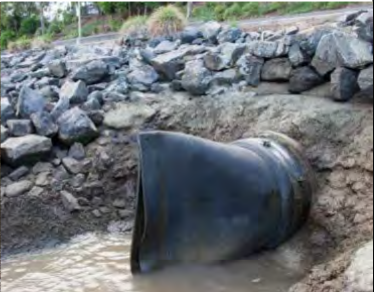
Photo 2. Example of a duck bill outlet structure
