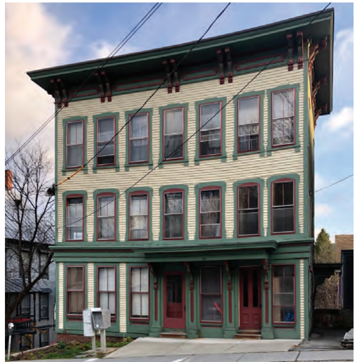
There are many excellent examples of multi-family multi-story housing in the historic downtowns of Vermont, this one in Montpelier, image credit: Susan Henderson
