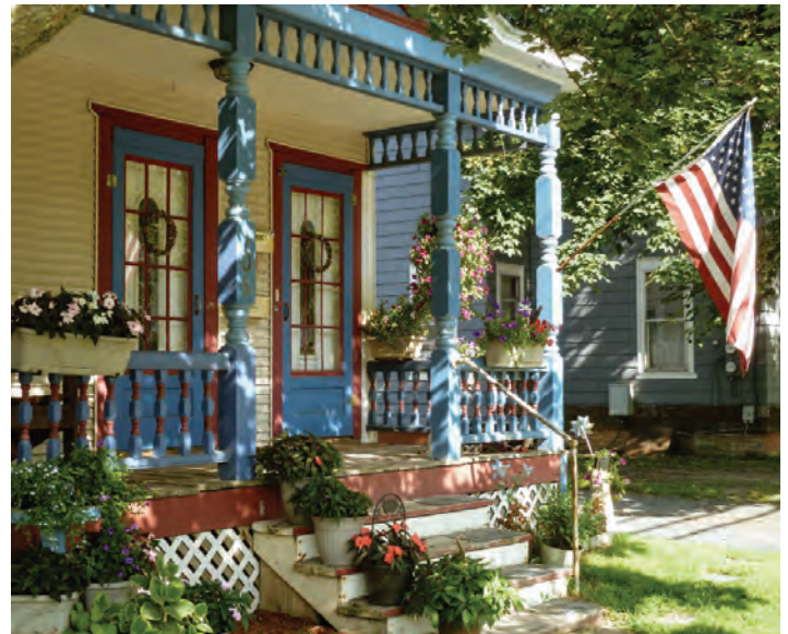
Duplex that fits into the neighborhood context in Waterbury, image credit: Richard Amore
