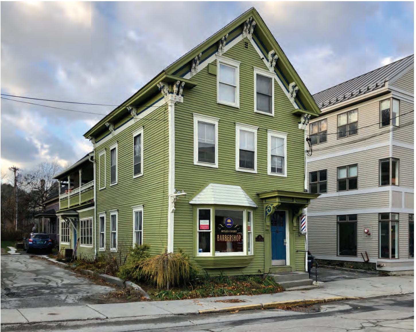
Live-work housing in Montpelier, image credit: Susan Henderson
