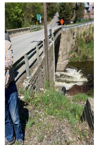
Bridge over the Lamoille River
