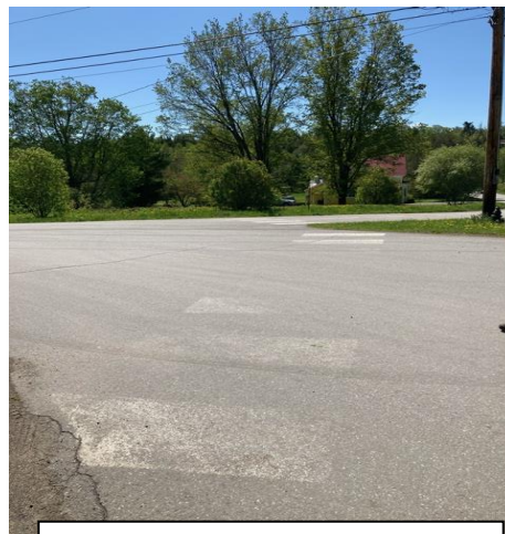
View across School Street intersection
