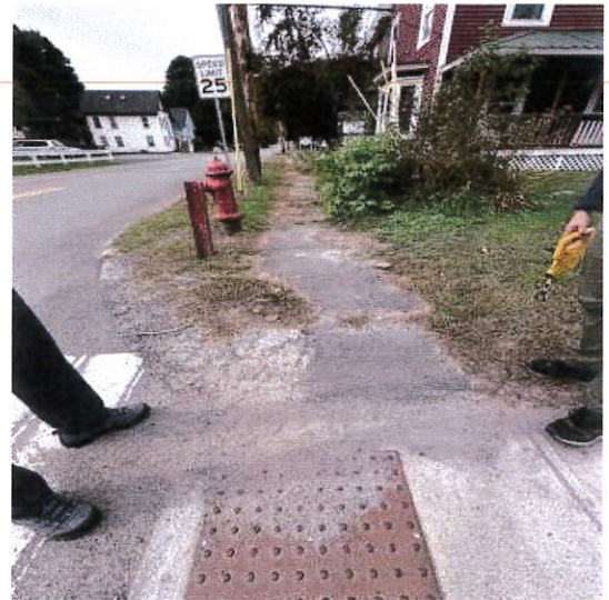
Intersection of Wolcott Street and Elm Street
