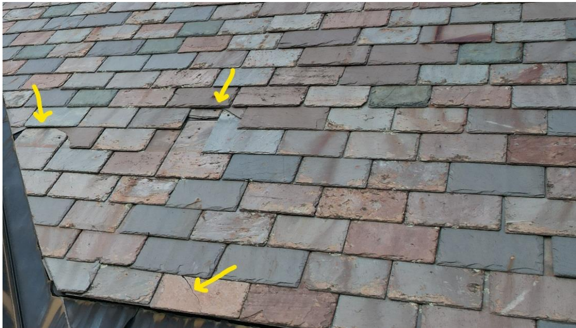
Hardwick Memorial Building – Missing, broken, and cracked slates at portico roof juncture (east).
