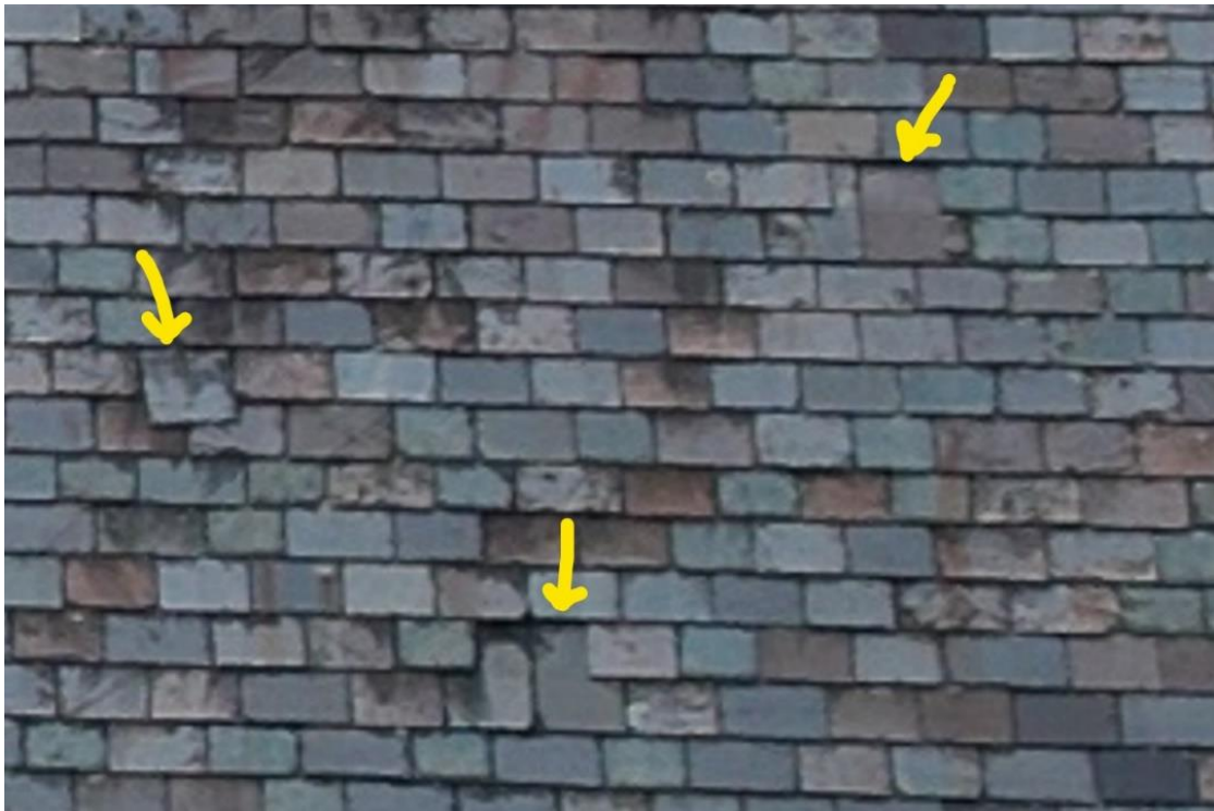
Hardwick Memorial Building – Loose and missing slates on SW roof surface.
