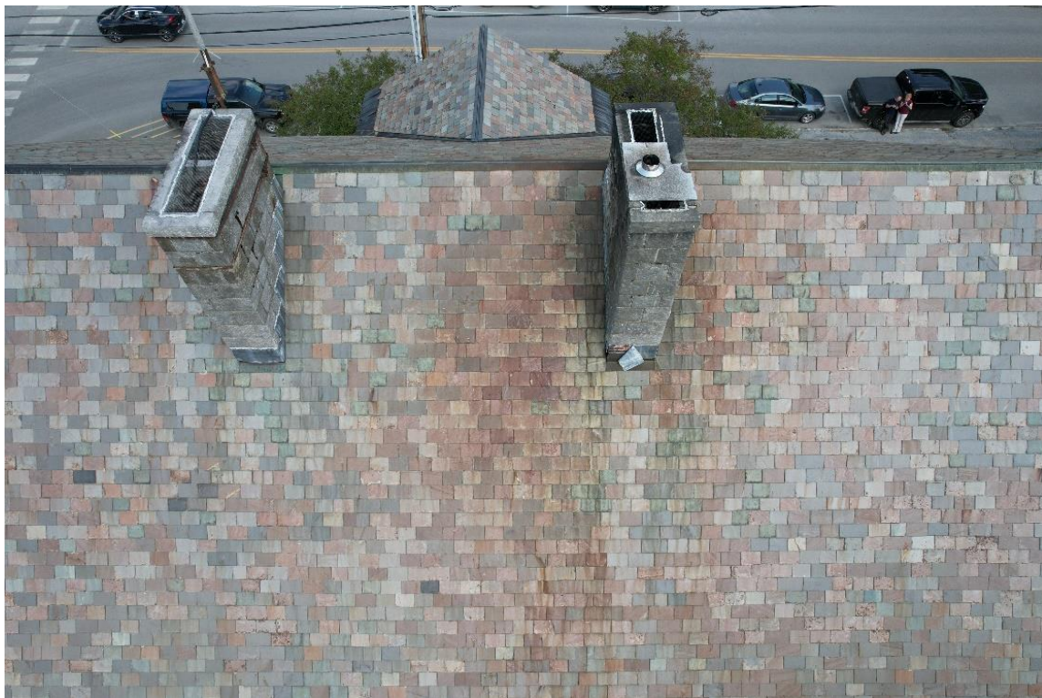
Hardwick Memorial Building - Damaged flashing at base of NE chimney.
