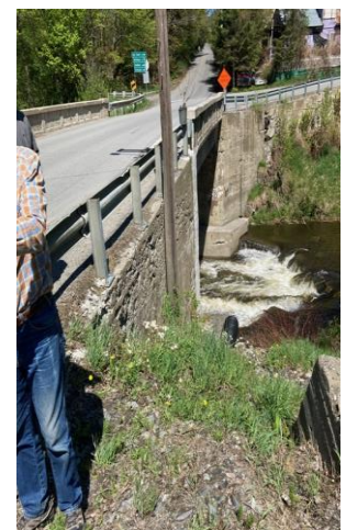
Bridge over the Lamoille River
