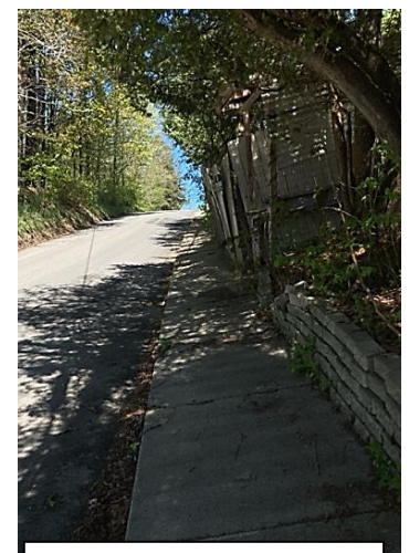
Uphill View of Brickhouse Rd
