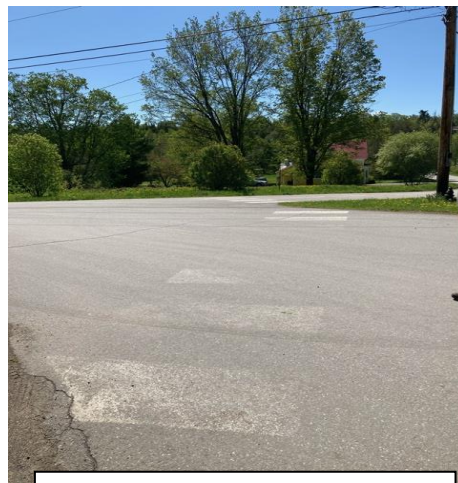
View across School Street intersection
