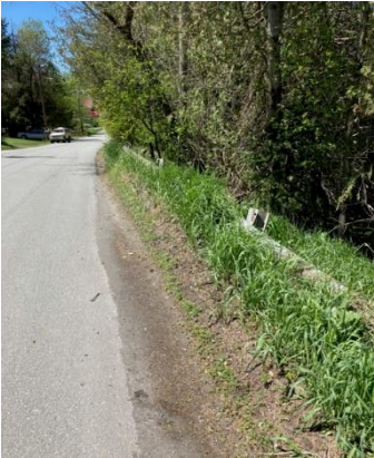
School Street embankment with dysfunctional guardrail
