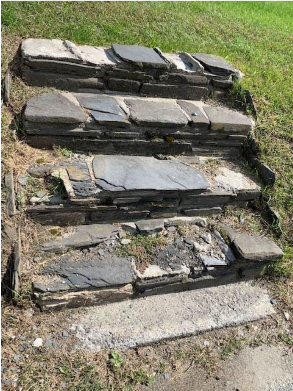
Image of stone steps at Memorial Park.
