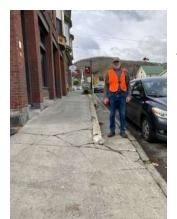
4) The south sidewalk splits into a two-level situation directly before the Holton Hill intersection. The upper level of the sidewalk has 6 ½ feet of width and then drops substantially and has an additional 2 feet.
