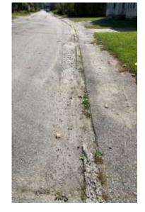
3) The sidewalk is continuous – no segments are missing. However, the sidewalk has a variety of angles and elevations which make walking difficult and virtually impossible to be utilized by a wheelchair or other form of mobility assistance.
