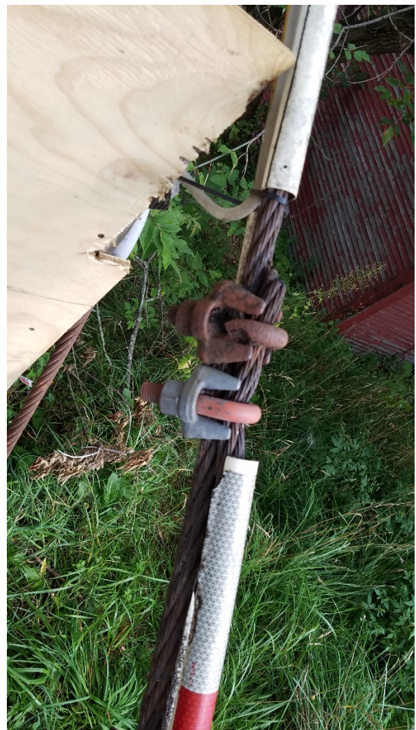
Photograph #2 – Cable clamp decay
