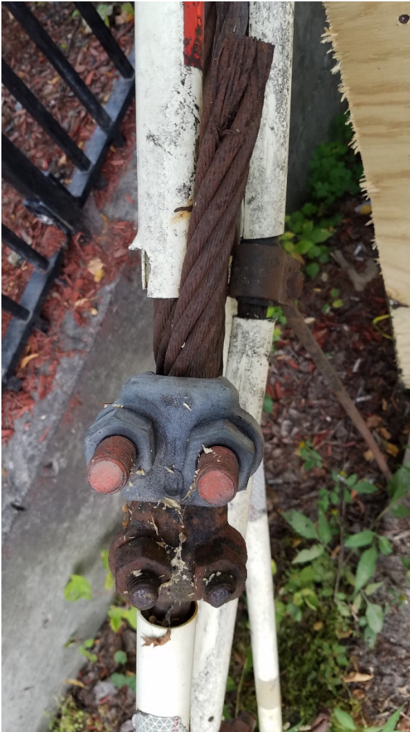
Photograph #1 – Cable clamp on backwards and less than recommended quantity
