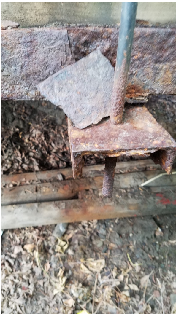
Photograph #4 – Deck Beam decay
