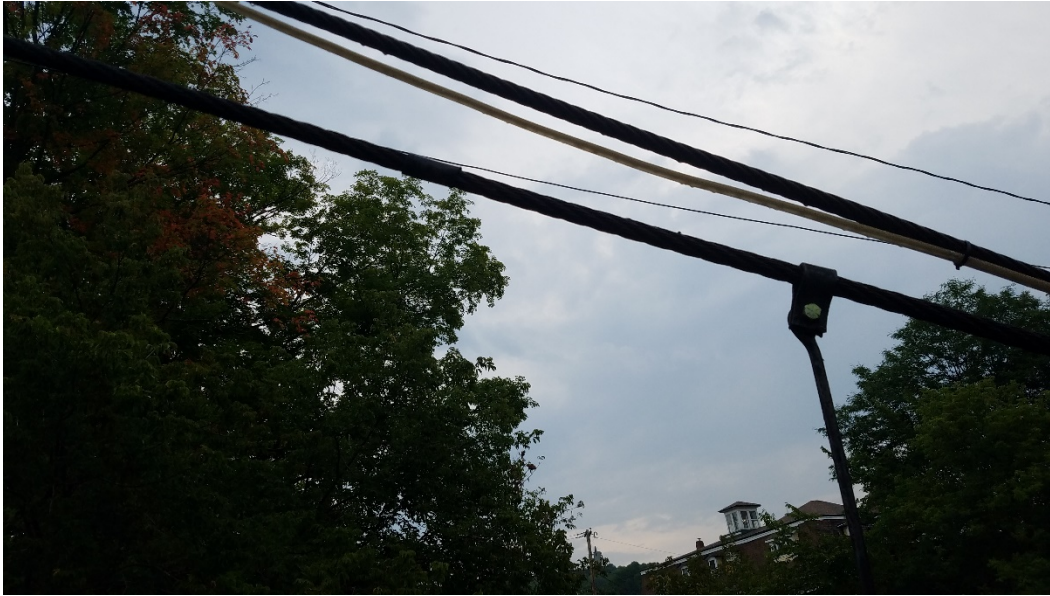
Photograph #3 – Drop cable slip
