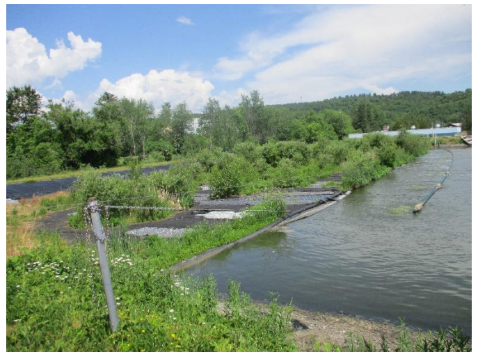
The Anaerobic Reactor Compartment (ARC) cover in Lagoon #1 is necessary to treat the wastewater produced by homes and businesses in Hardwick, but has deteriorated and is in need of replacement.
