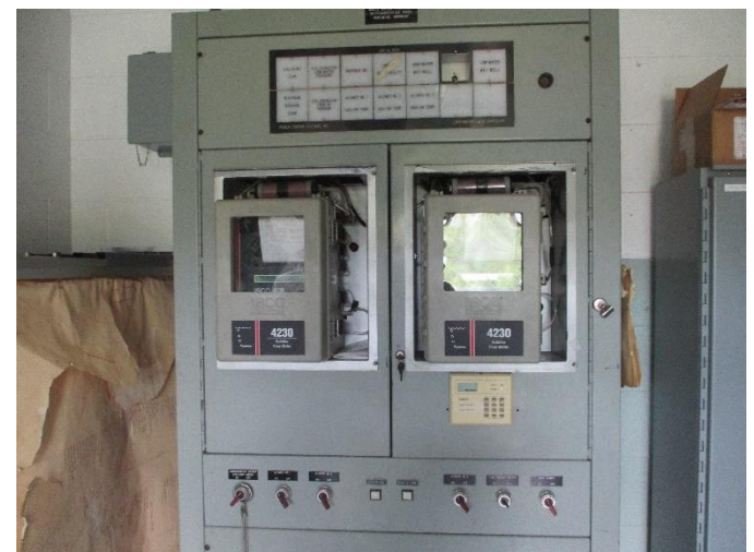
The project will improve the reliability of the facility by replacing outdated and deteriorating equipment, such as the 40-year-old control panel shown here.
