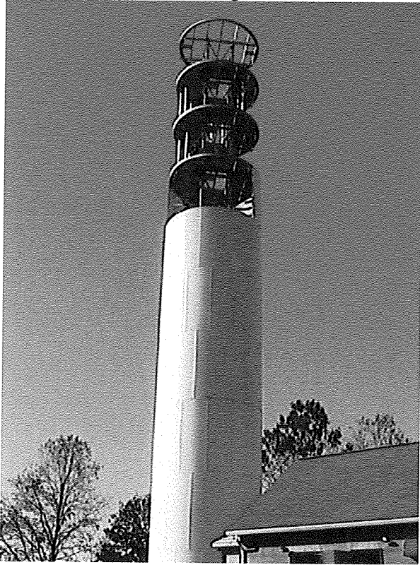
Hamden, CT - During Construction
