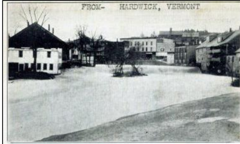
Hardwick, Vt.—Looking up toward Robie's dam from Wolcott St., November 4.
