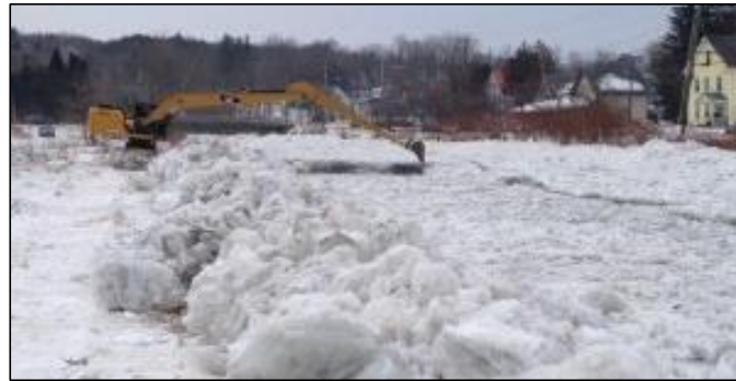
Long Reach Breaks Up Ice Jam in Hardwick (Copyright 2012 Tibbits Equipment Services, Inc. All Rights Reserved.)
